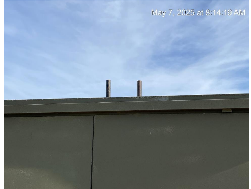
Relief vent risers caps missing
