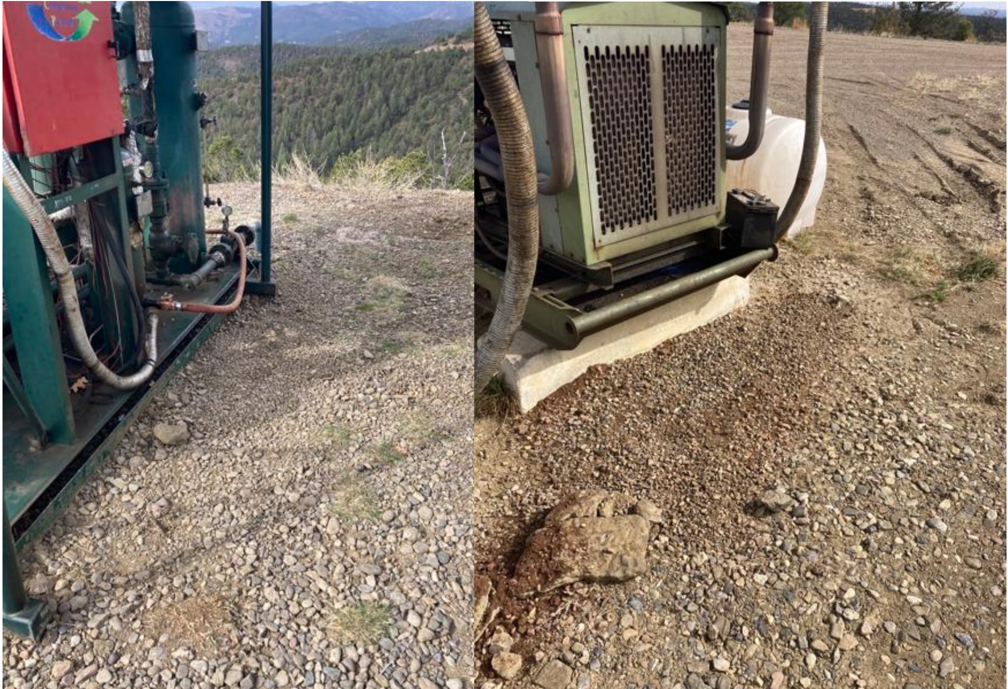
PHOTO 1: BOTH SKIDS HAVE BEEN CLEANED AND ALL OILY FLUIDS REMOVED. ALL OPERATING EQUIPMENT ON LOCATION HAS RECEIVED MECHANICAL MAINTENANCE. THE IMPACTED SOILS HAVE BEEN REMOVED AND THE SELF INSPECTION PROCESS REVIEWED.
