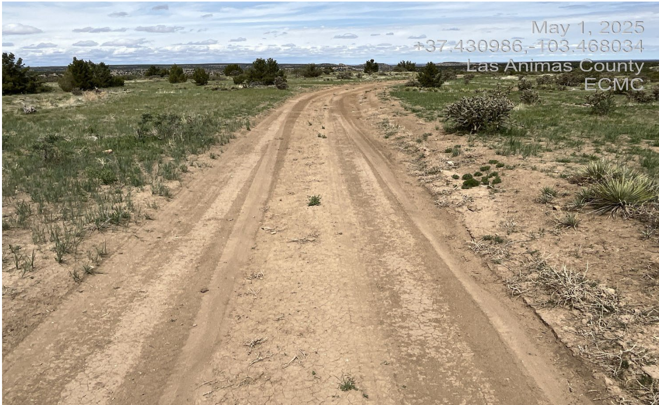
Photo 2. Facing north along the pre-existing access road near the location site. An access road will need to be built off of this road to the new location. Topsoil along the access road will need to be salvaged.
