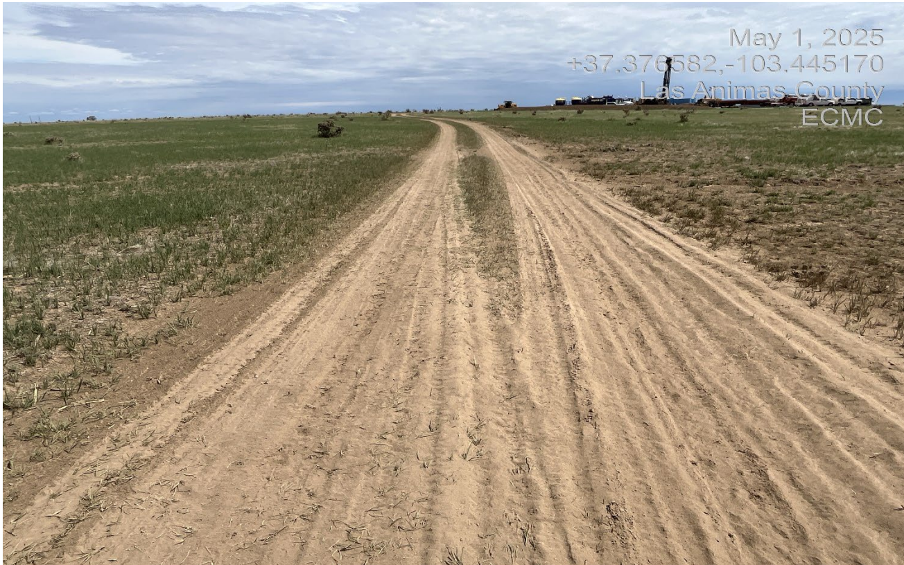
Photo 2. Facing north along the access road. The soils are very loose and susceptible to erosion.
