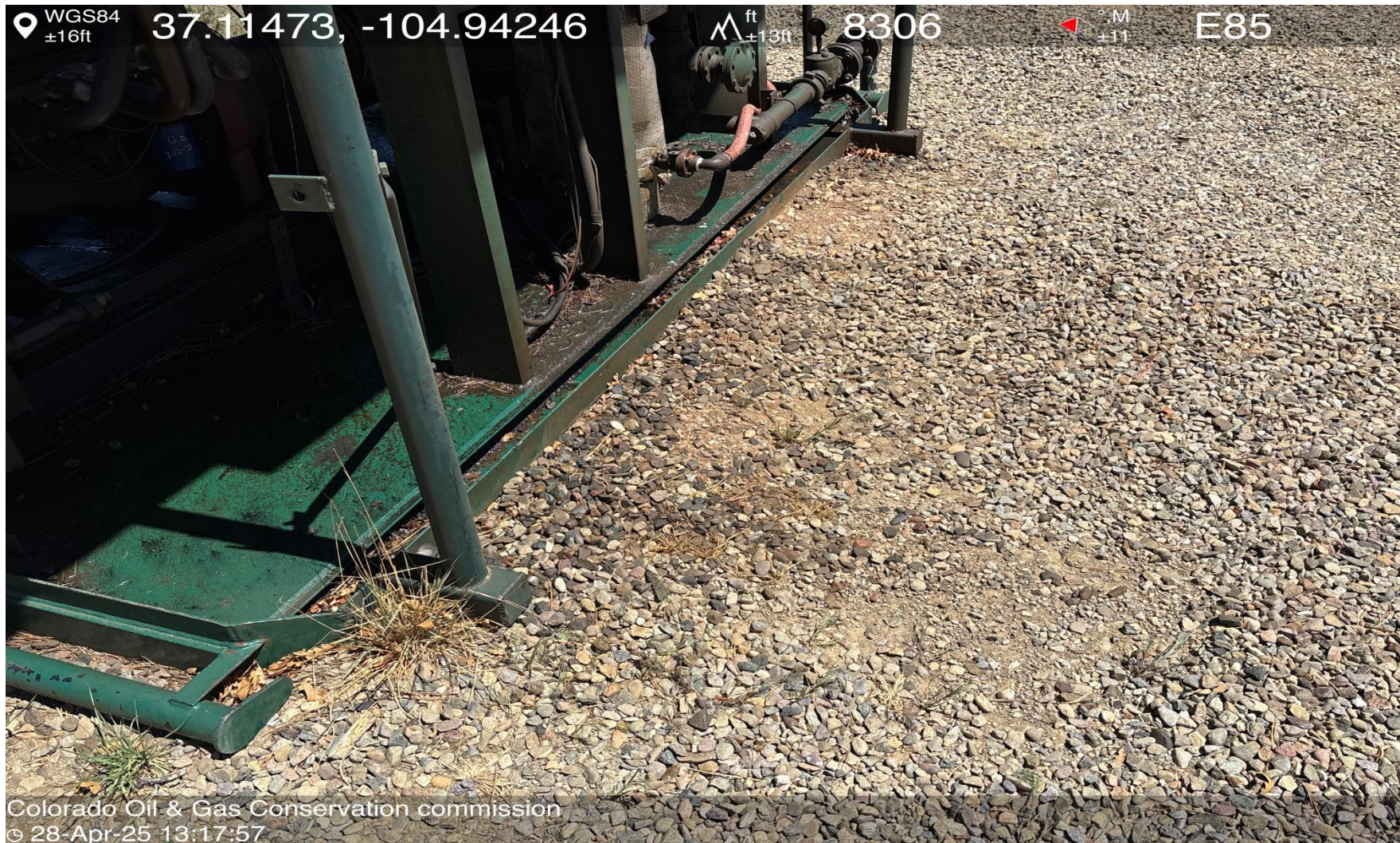
PHOTO 6: AREA OF IMPACTED SOIL NEAR COMPRESSOR SKID. Conduct maintenance on equipment, cleanup stained material and review self inspection processes. COMPLY WITH RULE 1002,(2).D. CA DATE 5-10-2025.
