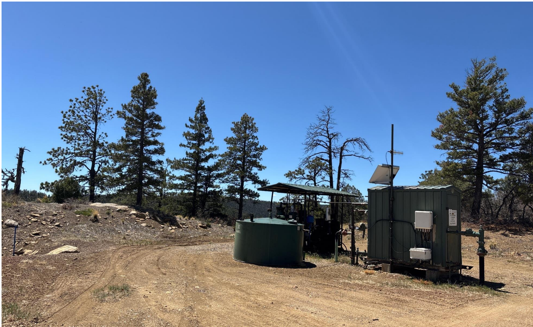
PHOTO 4: 25 BBL PRODUCED WATER TANK, COMPRESSOR AND METER HOUSE.
