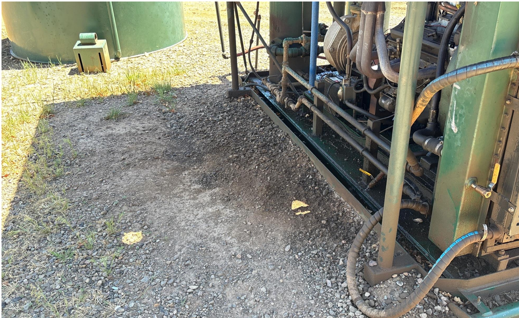
PHOTO 5: AREA OF IMPACTED SOIL NEAR COMPRESSOR SKID. Conduct maintenance on equipment, cleanup stained material and review self inspection processes. COMPLY WITH RULE 1002,.(2).D. CA DATE 5-10-2025.
