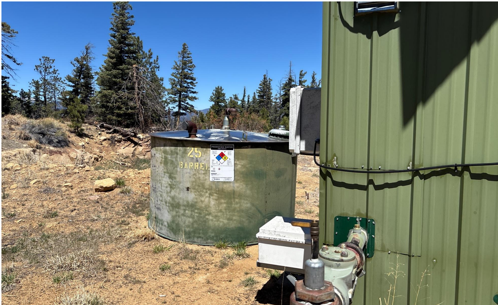
PHOTO 4: 25 BBL PRODUCED WATER TANK.
