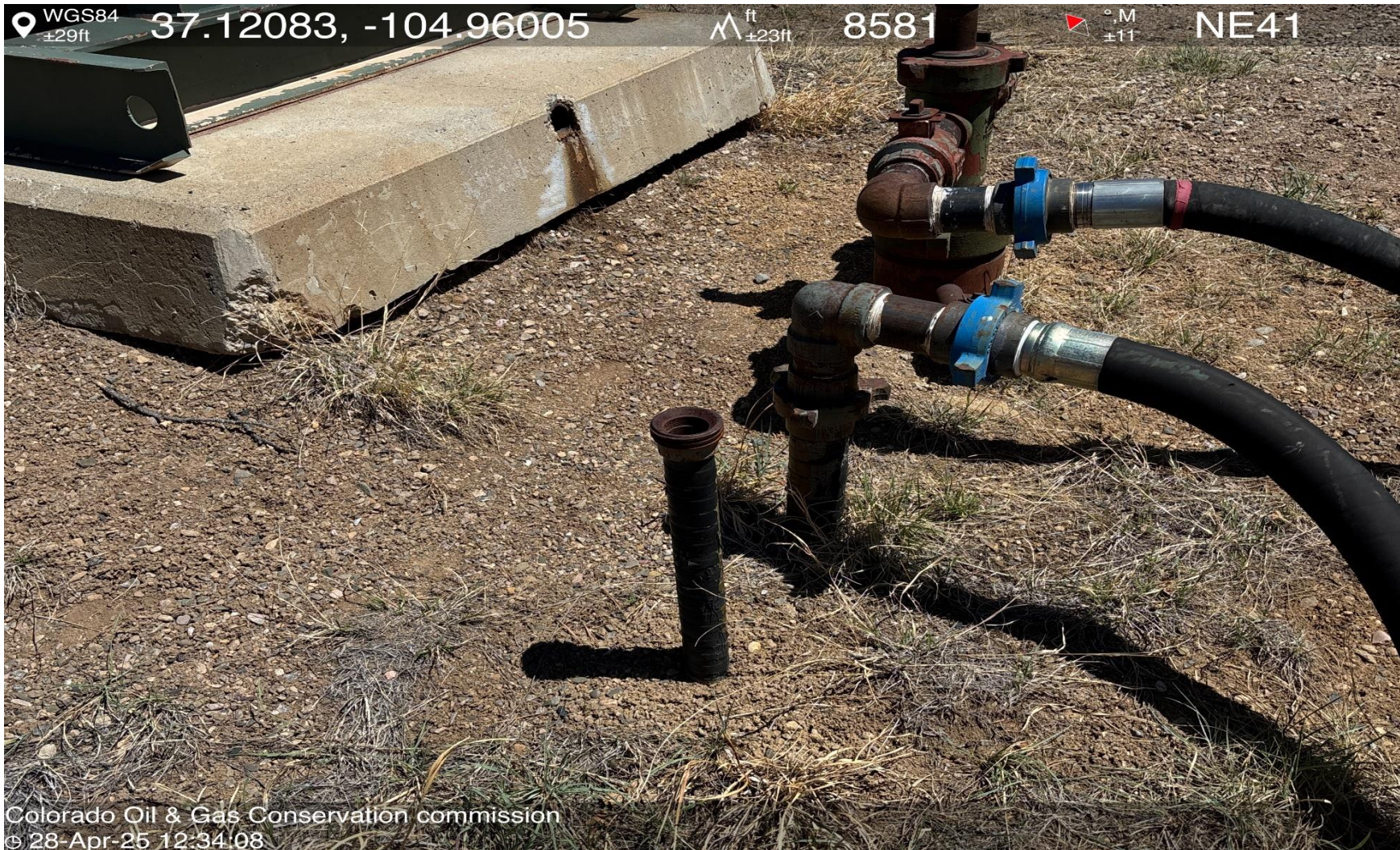
PHOTO 6: UNUSED EQUIPMENT ( 2" RISER BETWEEN WELLHEAD AND PUMPJACK NOT USED OR IDENTIFIED). REMOVE OR IDENTIFY/MARK ALL UNUSED RISERS PER RULE 606. CA DATE 5-9-2025.
