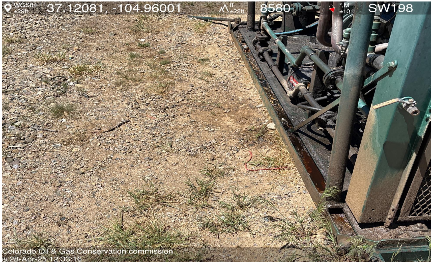
PHOTO 8: AREA OF IMPACTED SOIL NEAR COMPRESSOR. Conduct maintenance on equipment, cleanup stained material and review self inspection processes. COMPLY WITH RULE 1002,.(2).D. CA DATE 5-9-2025.
