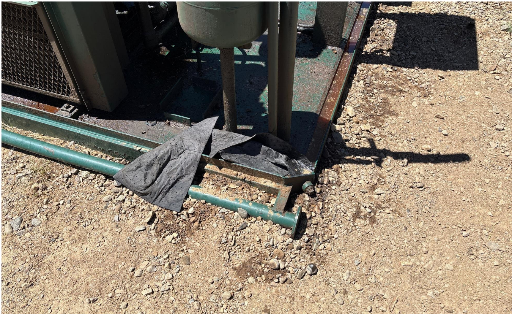
PHOTO 9: TRASH/ OILY WASTE INSIDE COMPRESSOR SKID WITHOUT NETTING. DRAIN OILY WASTE REPAIR ALL LEAKS AND REMOVE IMPACTED SOIL PER RULE 1002..(2).D & 1002.f.(2)B, Comply with general provisions of the oil and gas act for wildlife protection AND SB-181. CA DATE 4-29-2025.
