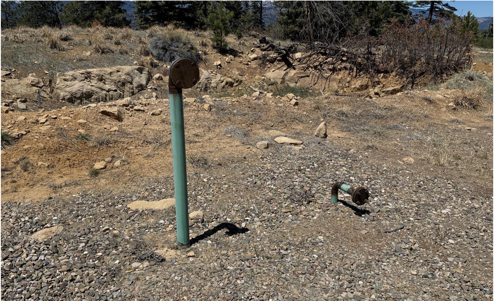
PHOTO 5: UNUSED EQUIPMENT ( A 3" RISER AND A 2" RISER BETWEEN WELLHEAD AND METERHOUSE NOT USED OR IDENTIFIED). REMOVE OR IDENTIFY/MARK ALL UNUSED RISERS PER RULE 606. CA DATE 5-9-2025.
