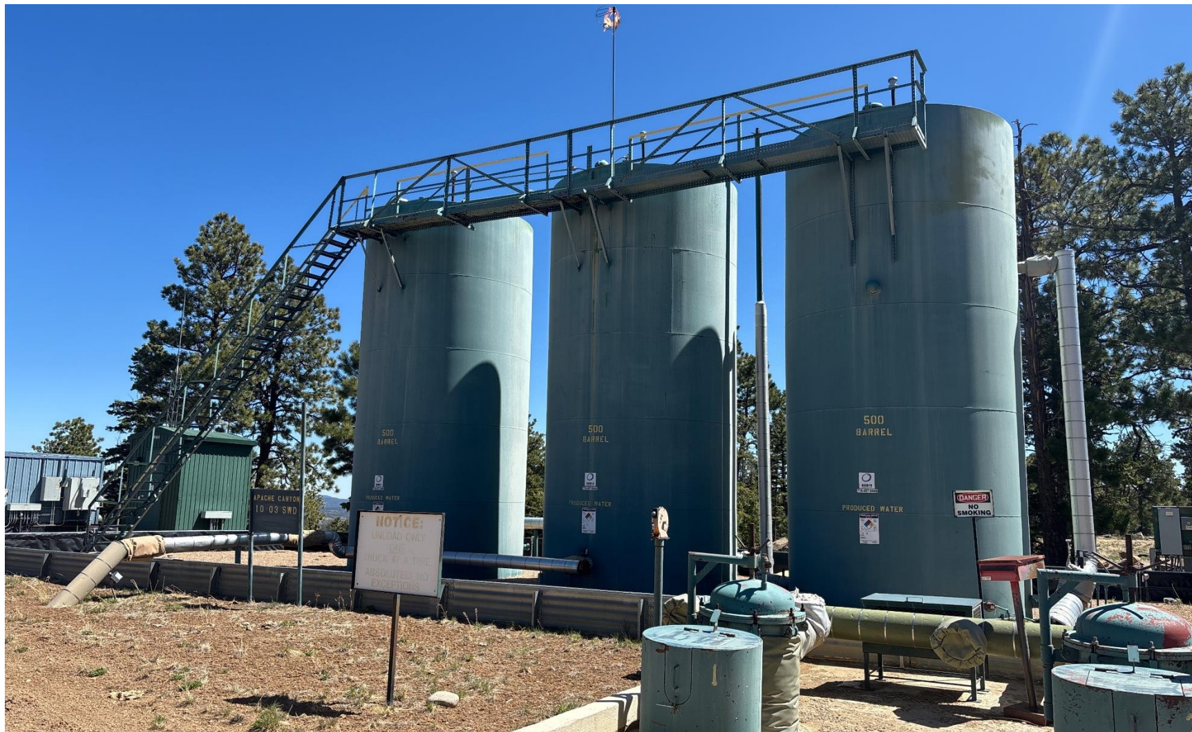
PHOTO 4: PRODUCED WATER TANK BATTERY.
