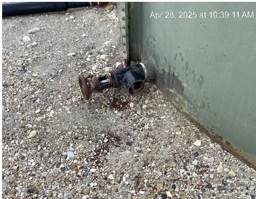
Covered staining. Open end tank valve.
