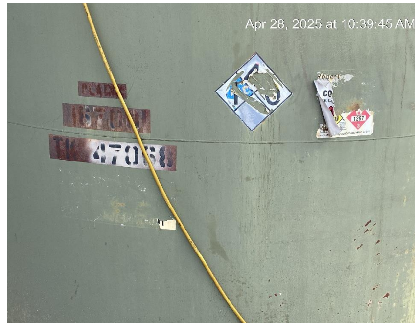
Damaged and incomplete tank labels
