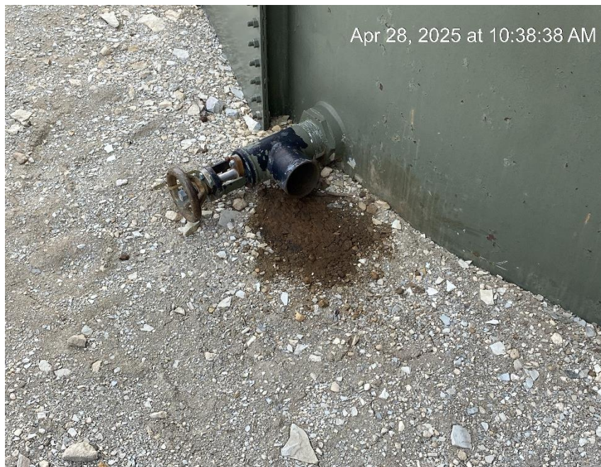
Open end tank valve. Oily waste and stained soil.
