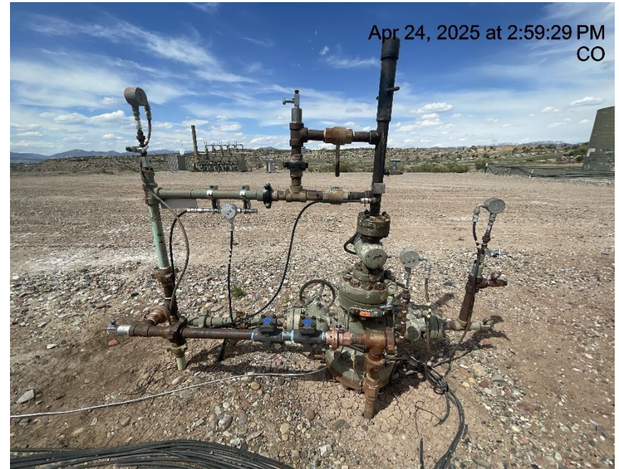
Photo # 6123 BOULTON 33-6 BH line tied into flowline & also tied into separator at the A valve bypass
