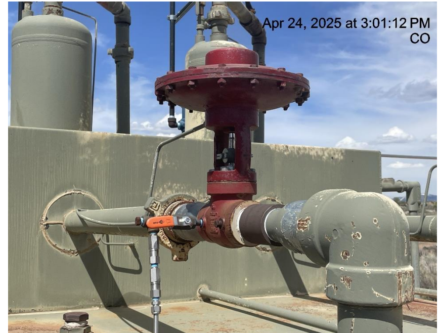
Photo # 6128 BOULTON 33-6 BH line tied into separator at the A valve bypass
