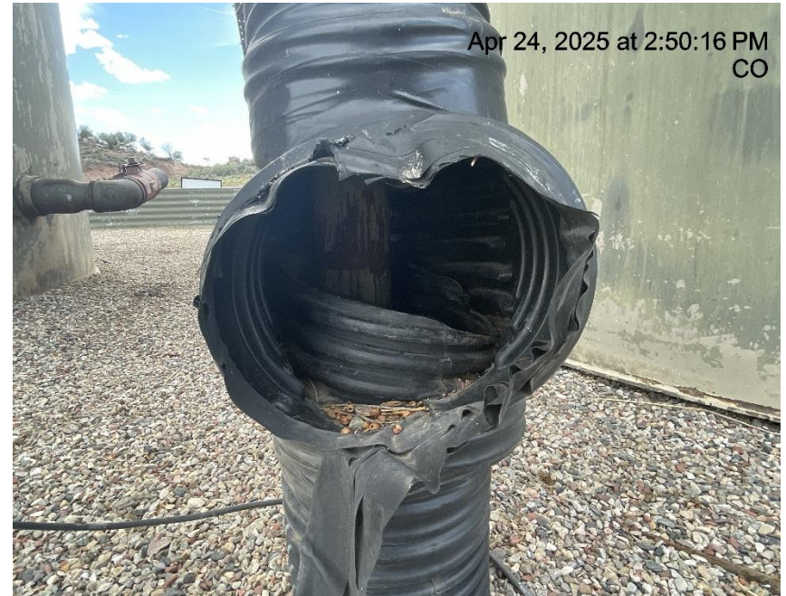
Photo # 6121 Flowline heating insulation open ended /wildlife hazard/available for entry by wildlife
