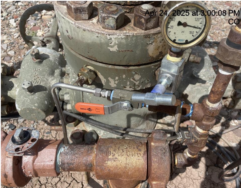
Photo # 6126 BOULTON 33-6 BH line tied into separator at the A valve bypass
