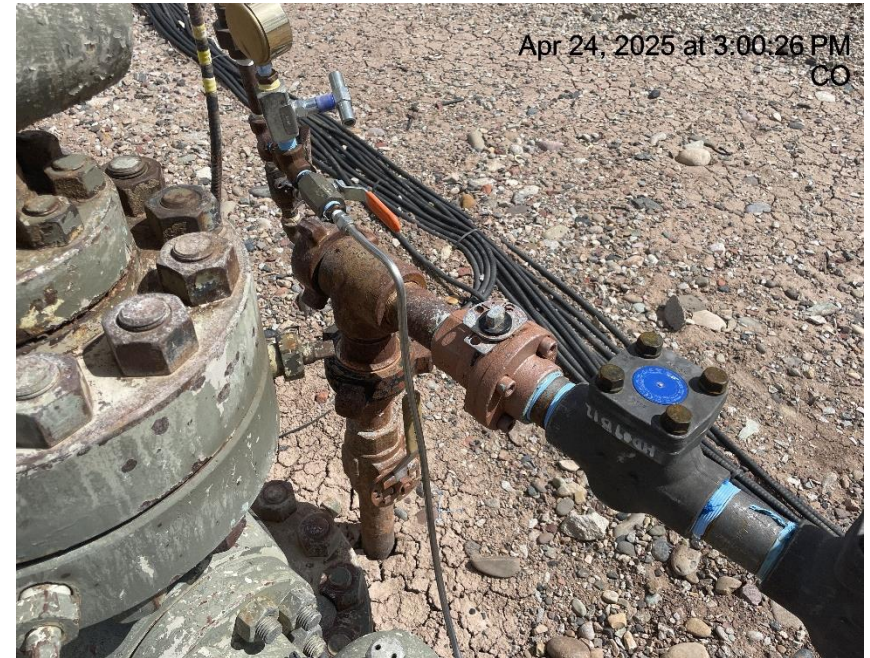
Photo # 6127 BOULTON 33-6 BH line tied into separator at the A valve bypass
