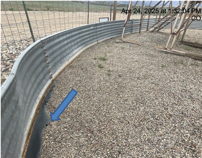
Photo # 5678 Hole in liner/liner needs maintenance
