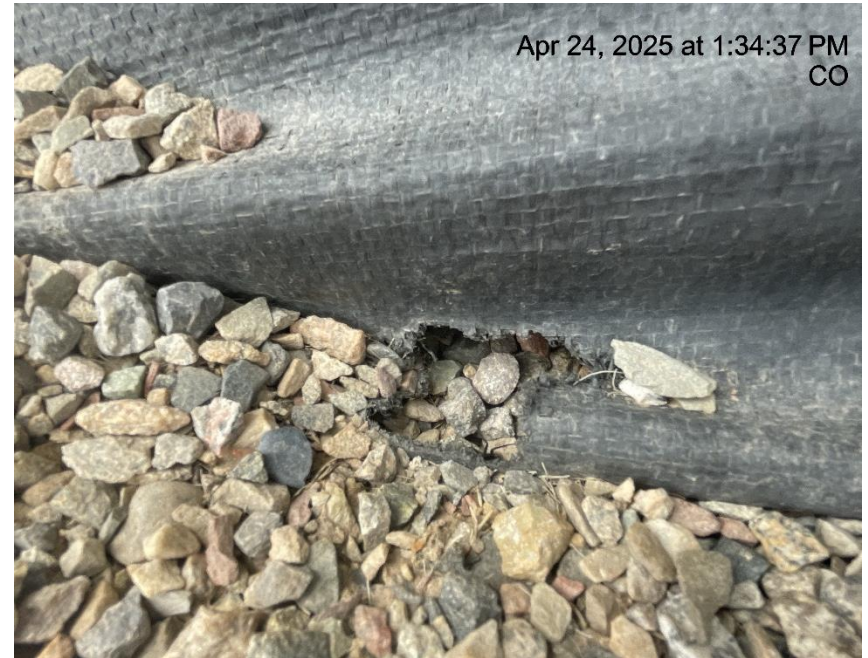
Photo # 5681 Hole in liner/liner needs maintenance
