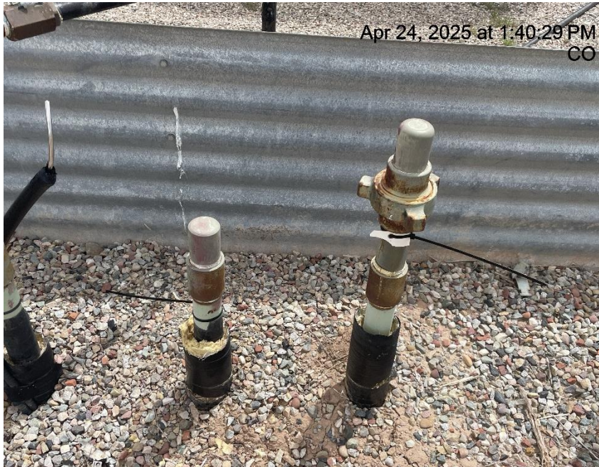
Photo # 5672 Unused flowlines lack lockout tagout (OOSLAT)
