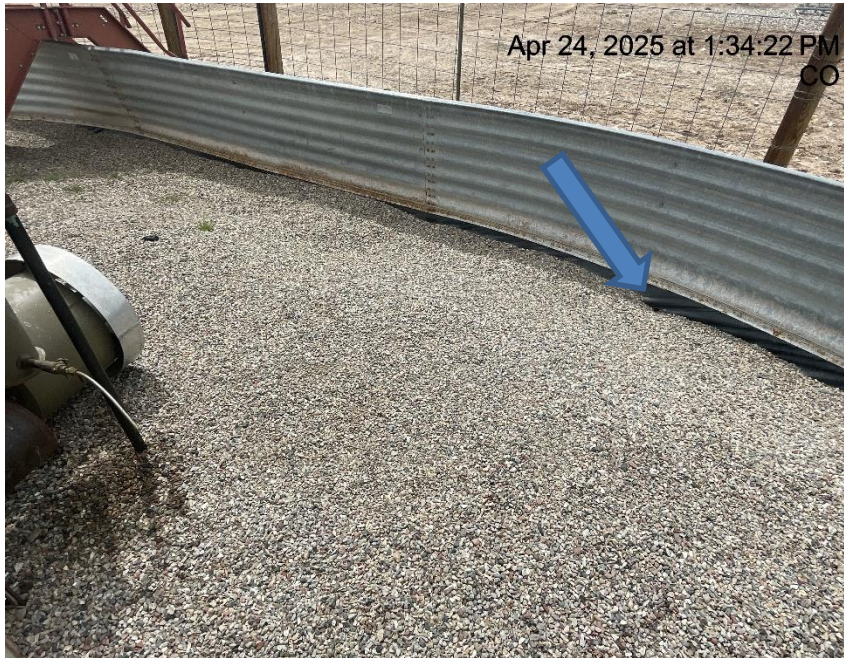
Photo # 5680 Hole in liner/liner needs maintenance
