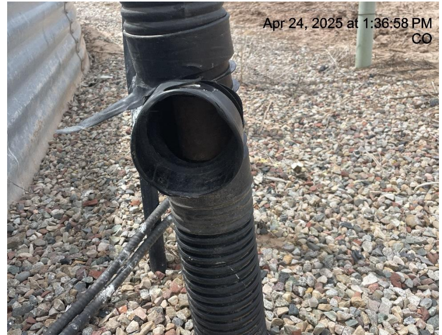
Photo # 5677 Flowline heating insulation open ended /wildlife hazard/available for entry by wildlife
