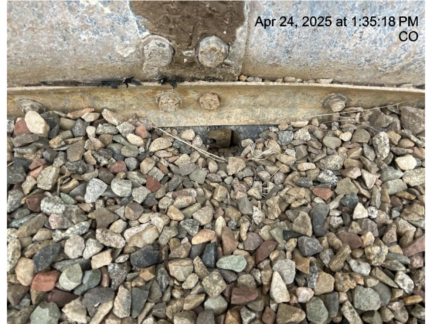
Photo # 5683 Hole in liner/liner needs maintenance
