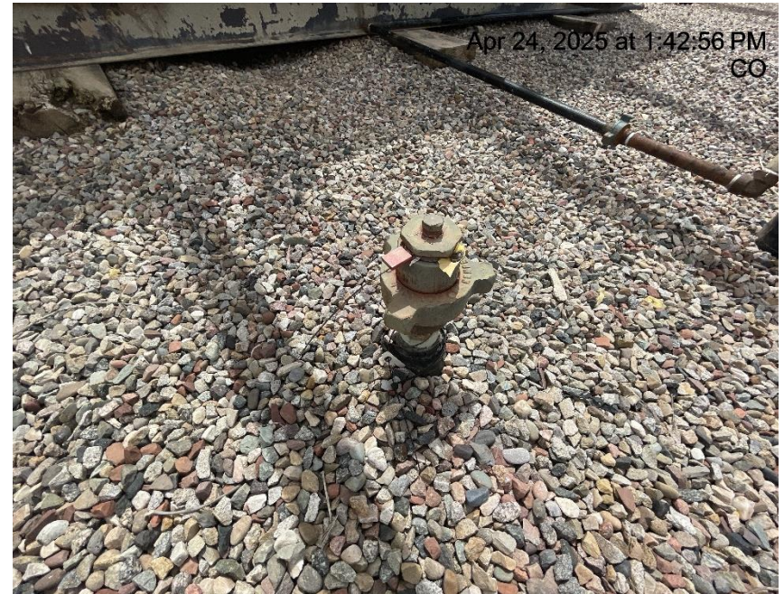
Photo # 5673 Unused flowline lacks lockout tagout (OOSLAT)
