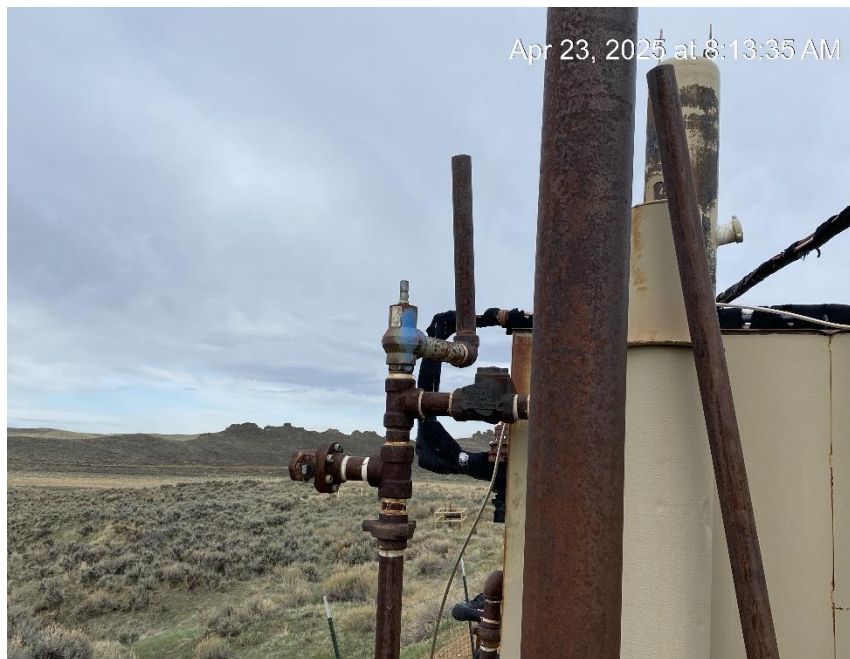
Unprotected relief vent riser
