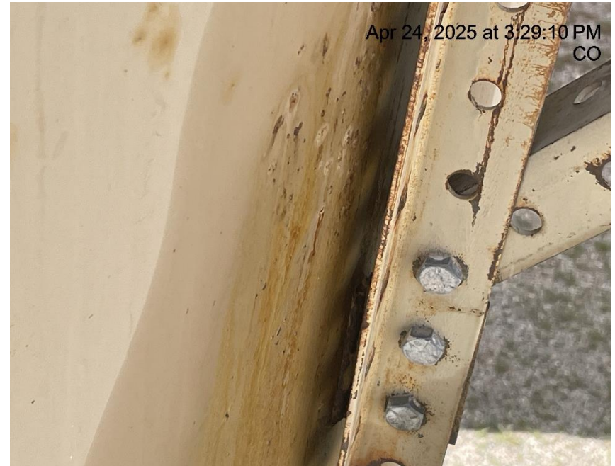
Photo # 6259 Possible tank failure - Suspected leak on production tank/tank appears to lack integrity
