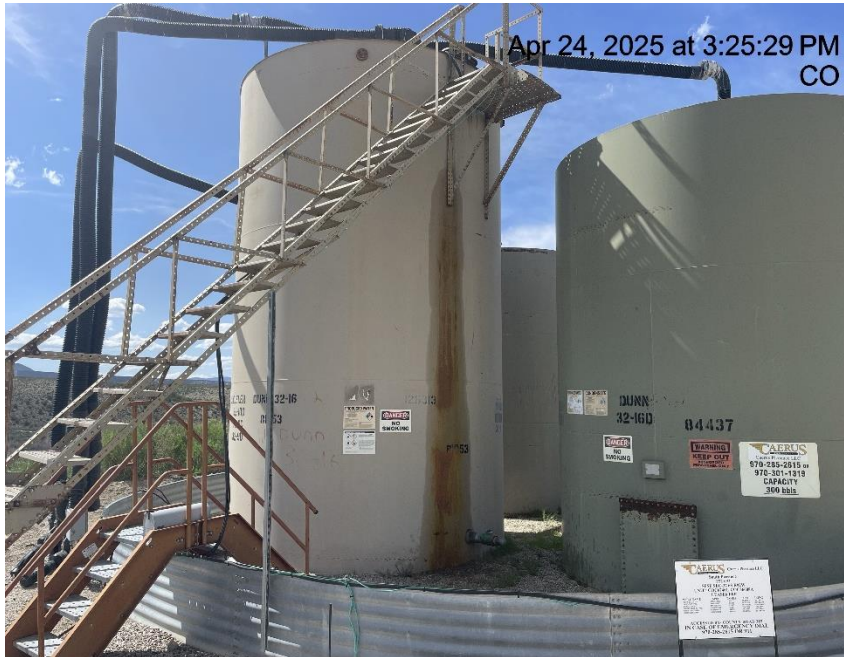
Photo # 6254 Possible tank failure - Suspected leak on production tank/tank appears to lack integrity
