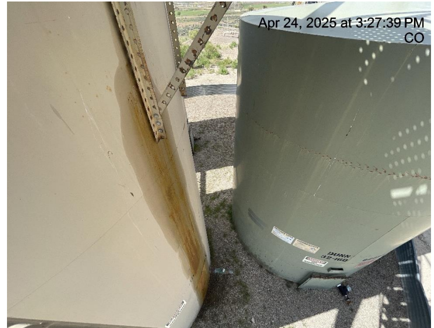
Photo # 6263 Possible tank failure - Suspected leak on production tank/tank appears to lack integrity
