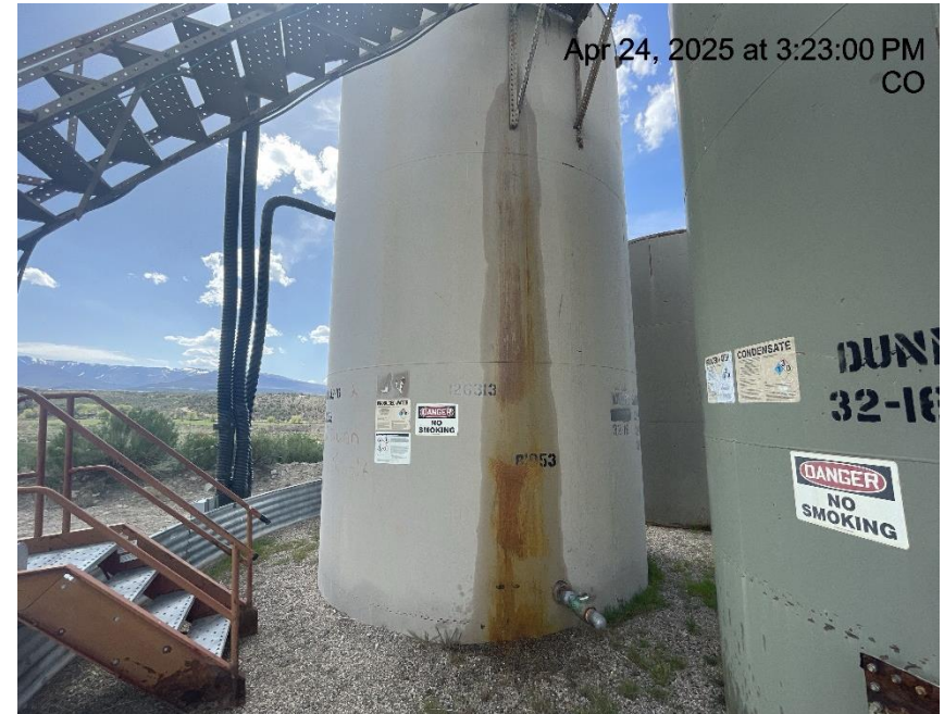
Photo # 6255 Possible tank failure - Suspected leak on production tank/tank appears to lack integrity
