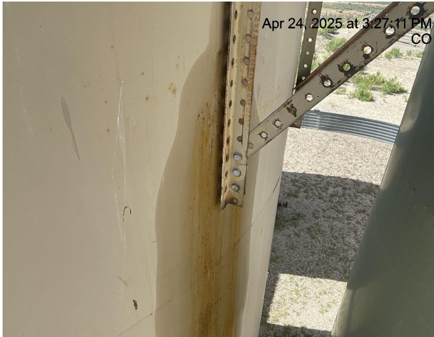
Photo # 6262 Possible tank failure - Suspected leak on production tank/tank appears to lack integrity
