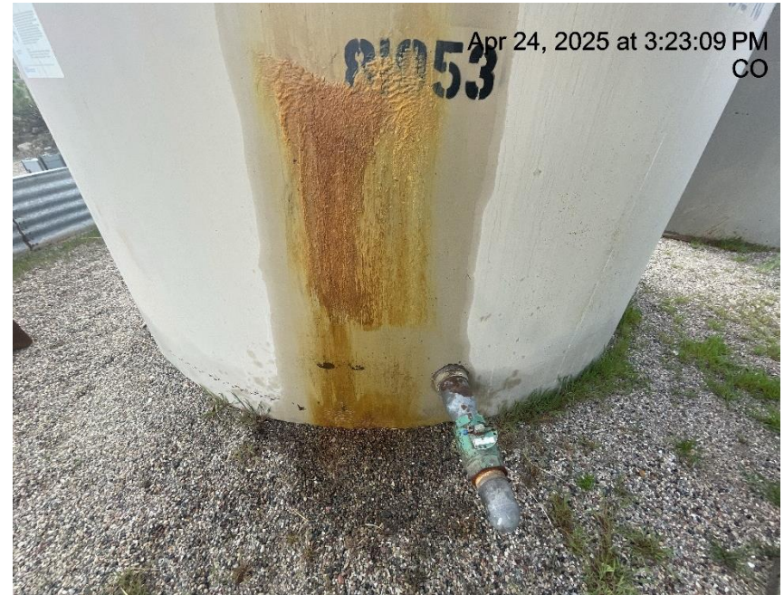
Photo # 6267 Possible tank failure - Suspected leak on production tank/tank appears to lack integrity
