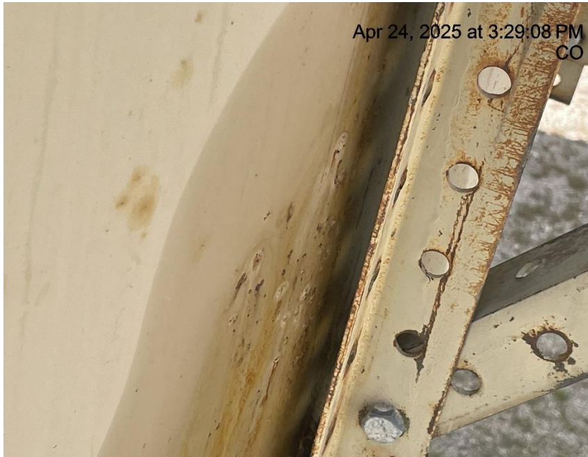
Photo # 6258 Possible tank failure - Suspected leak on production tank/tank appears to lack integrity
