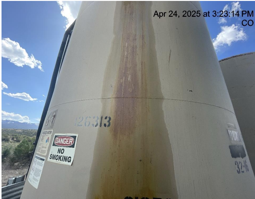
Photo # 6266 Possible tank failure - Suspected leak on production tank/tank appears to lack integrity
