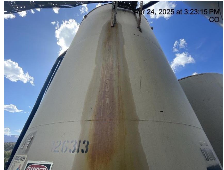
Photo # 6265 Possible tank failure - Suspected leak on production tank/tank appears to lack integrity
