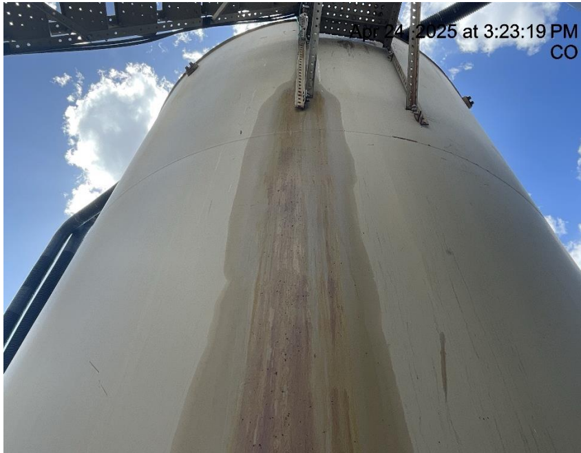
Photo # 6264 Possible tank failure - Suspected leak on production tank/tank appears to lack integrity
