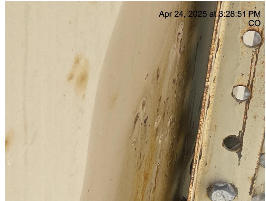
Photo # 6261 Possible tank failure - Suspected leak on production tank/tank appears to lack integrity
