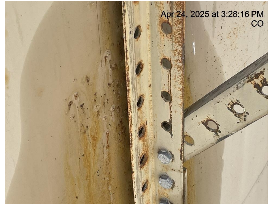
Photo # 6257 Possible tank failure - Suspected leak on production tank/tank appears to lack integrity
