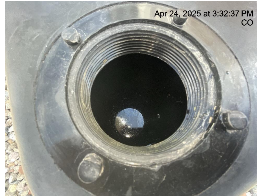
6269 Failure to maintain chemical BMP – Chemical tank containment approximately 2/3 full of fluid/BMP insufficient to contain possible spill
