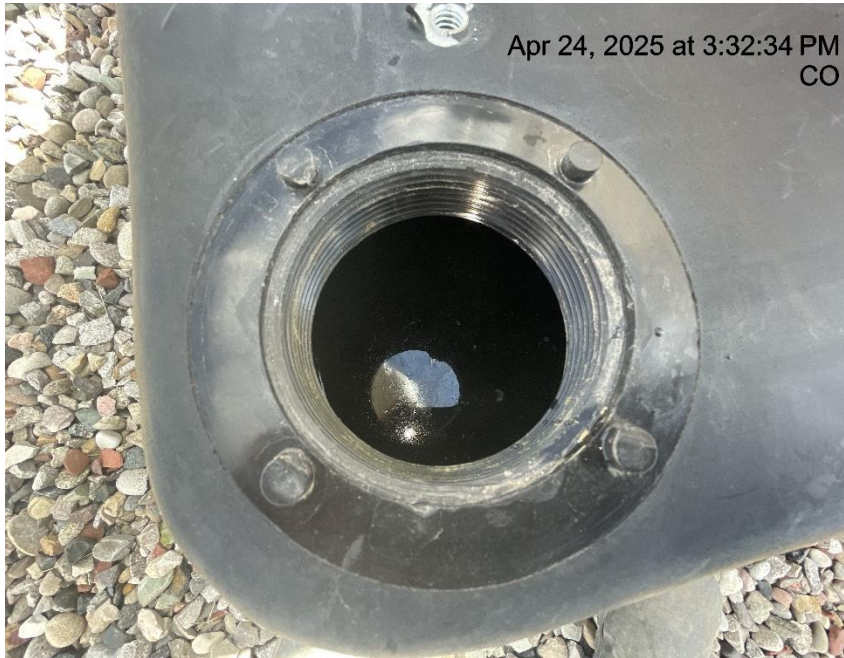
Photo # 6268 Failure to maintain chemical BMP – Chemical tank containment approximately 2/3 full of fluid/BMP insufficient to contain possible spill
