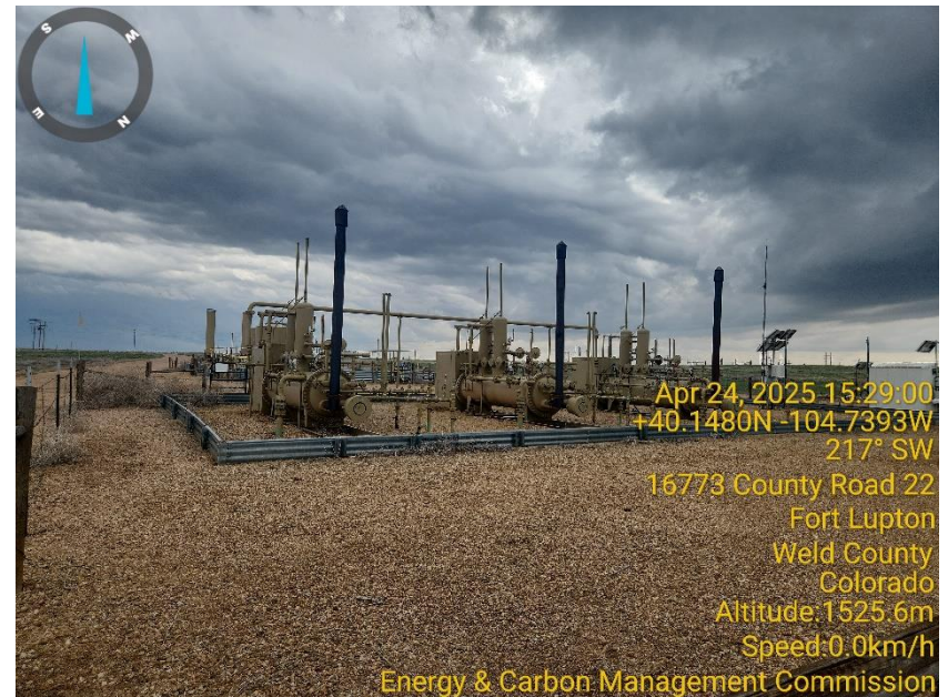
Photo 6 Horizontal Heated Separators.
