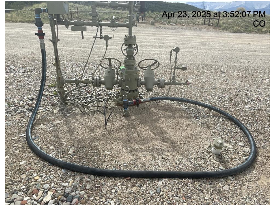
Photo # 5267 No check valve on line connecting BH line to flowline Benjamin Federal 33-4B (K28NW) well
