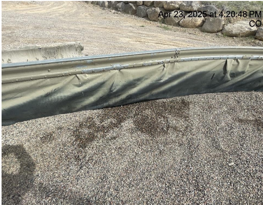
Photo # 5262 Staining in secondary containment
