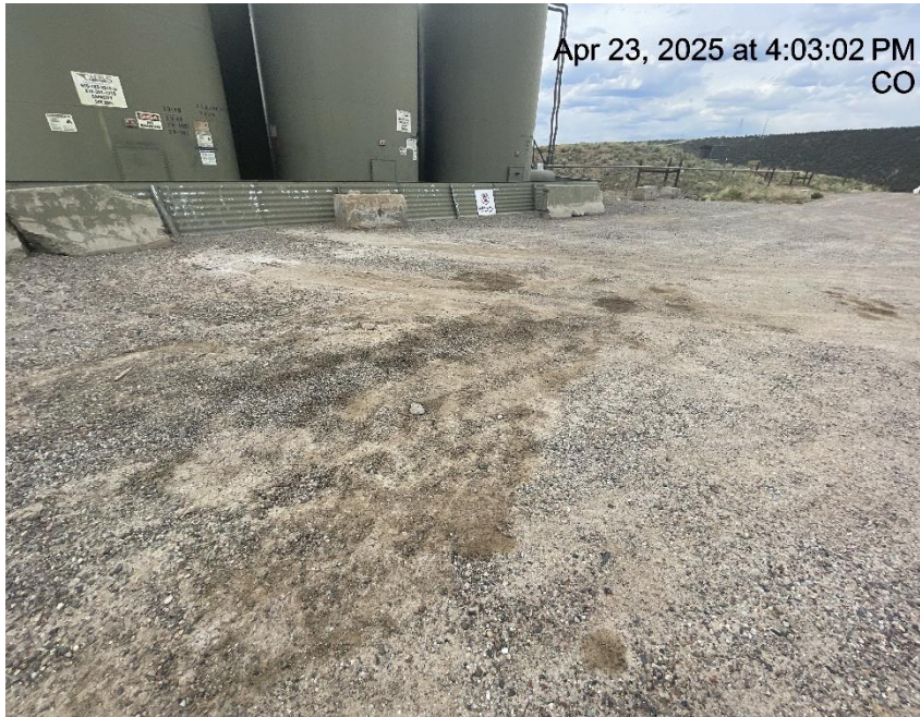
Photo # 5254 Staining near tank battery
