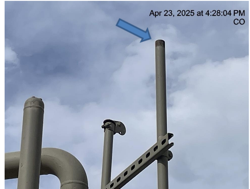
Photo # 5251 PRV vent line does not comply with CECMC pressure safety device rules
