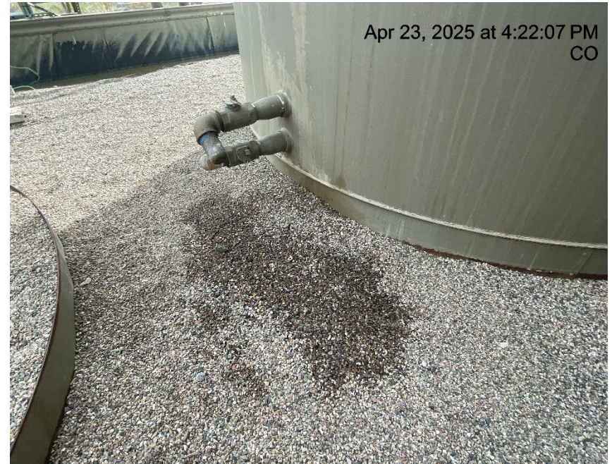
Photo # 5263 Staining in secondary containment
