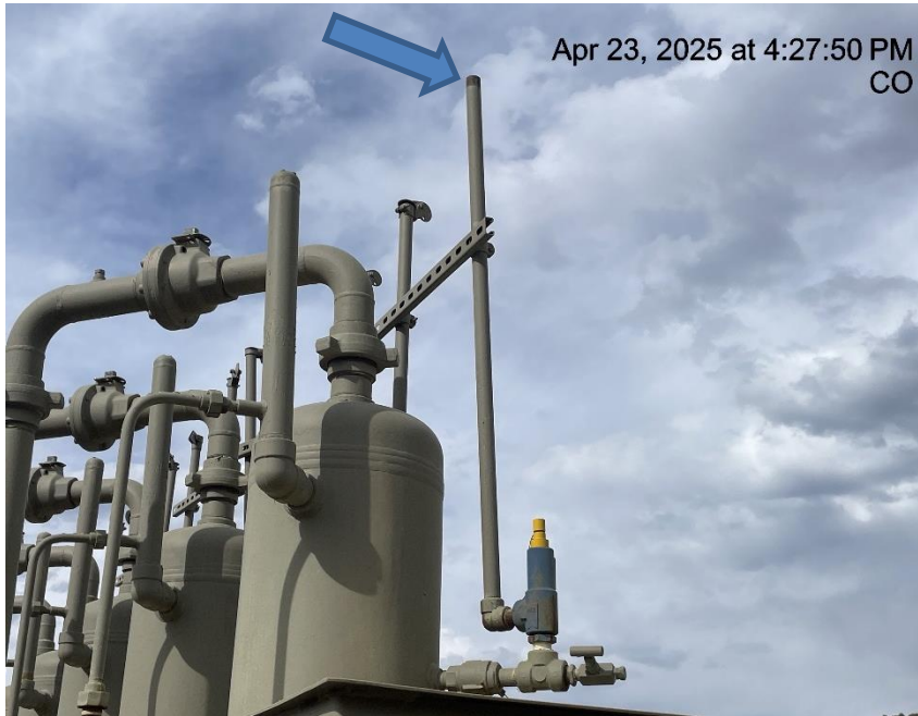
Photo # 5250 PRV vent line does not comply with CECMC pressure safety device rules
