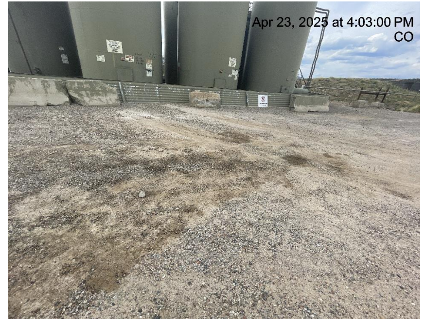
Photo # 5253 Staining near tank battery
