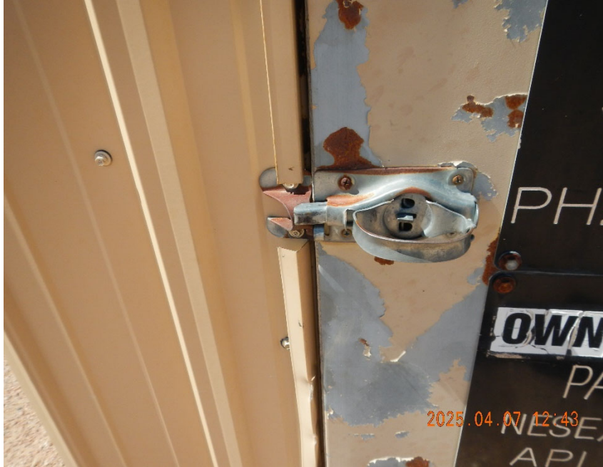
5. Broken door handle on meter shed door. Door is jammed shut.
