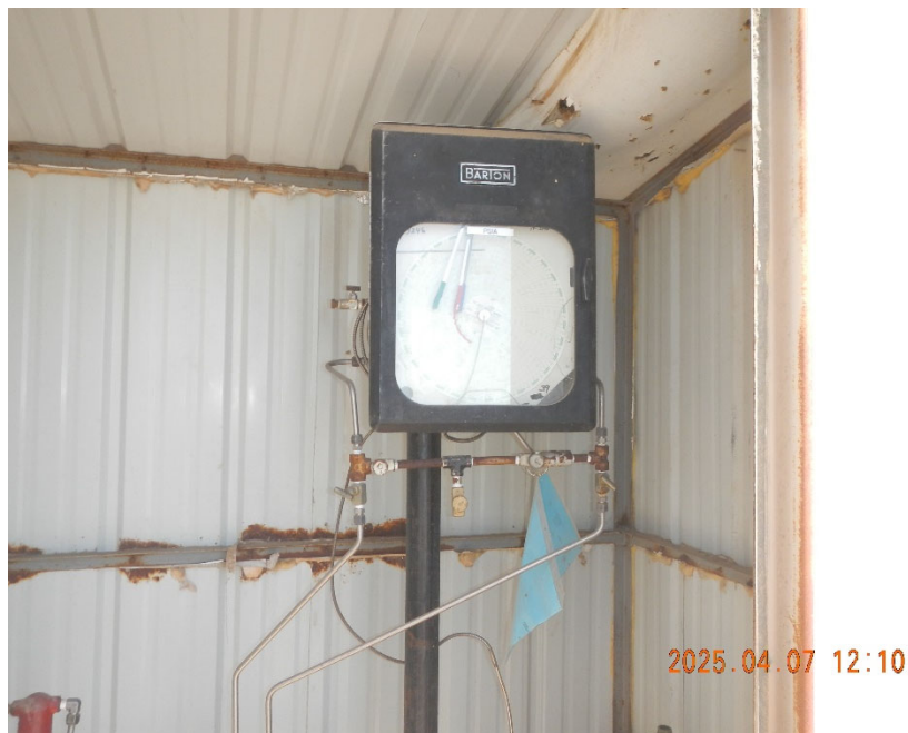
5. Gas meter inside meter shed.
