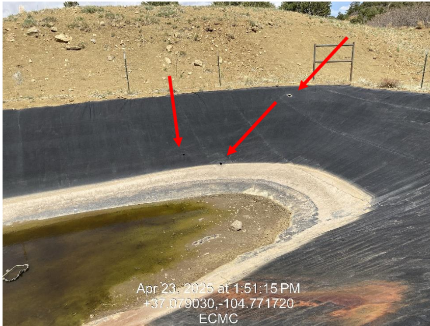
Photo 5 – Holes in liner
