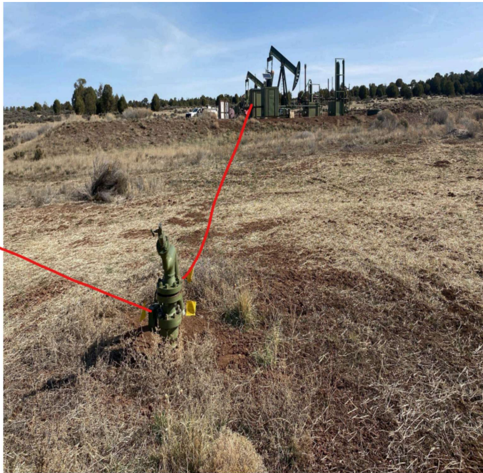
Photo 4. Gas line riser that remains in the northwest corner of the pi
