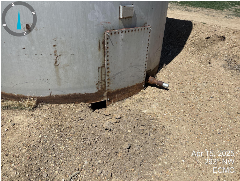
Photo 3. Looking at the east side of the northern tank. Animal holes are present underneath the tank.
