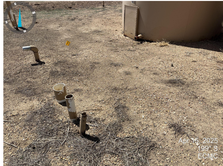
Photo 4. Photo taken on the east side of location. PVC pipes behind the tanks do not have wildlife exclusion devices installed.
