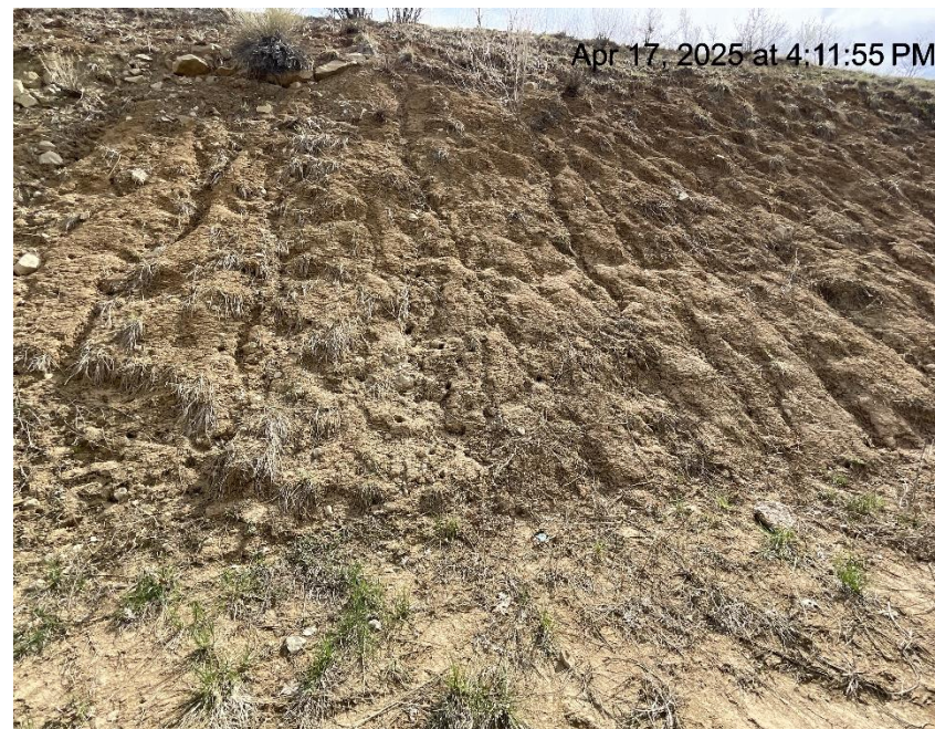
Photo # 3332 Erosion & transport of sediment on cut slope /insufficient BMP's
