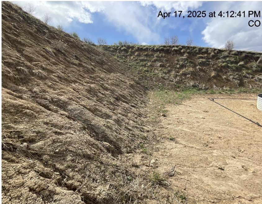
Photo # 3335 Erosion & transport of sediment on cut slope /insufficient BMP's
