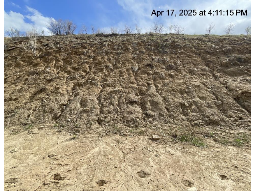
Photo # 3334 Erosion & transport of sediment on cut slope /insufficient BMP's
