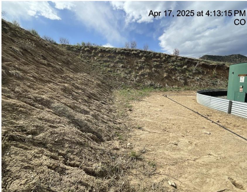
Photo # 3337 Erosion & transport of sediment on cut slope /insufficient BMP's
