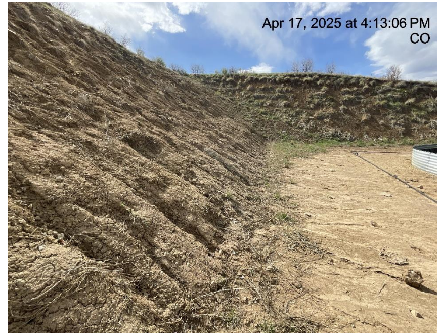
Photo # 3336 Erosion & transport of sediment on cut slope /insufficient BMP's
