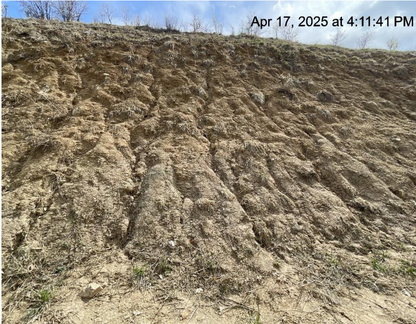
Photo # 3333 Erosion & transport of sediment on cut slope /insufficient BMP's
