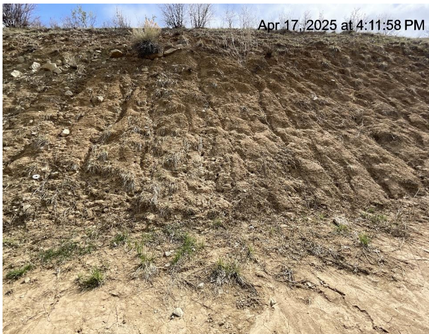
Photo # 3331 Erosion & transport of sediment on cut slope /insufficient BMP's
