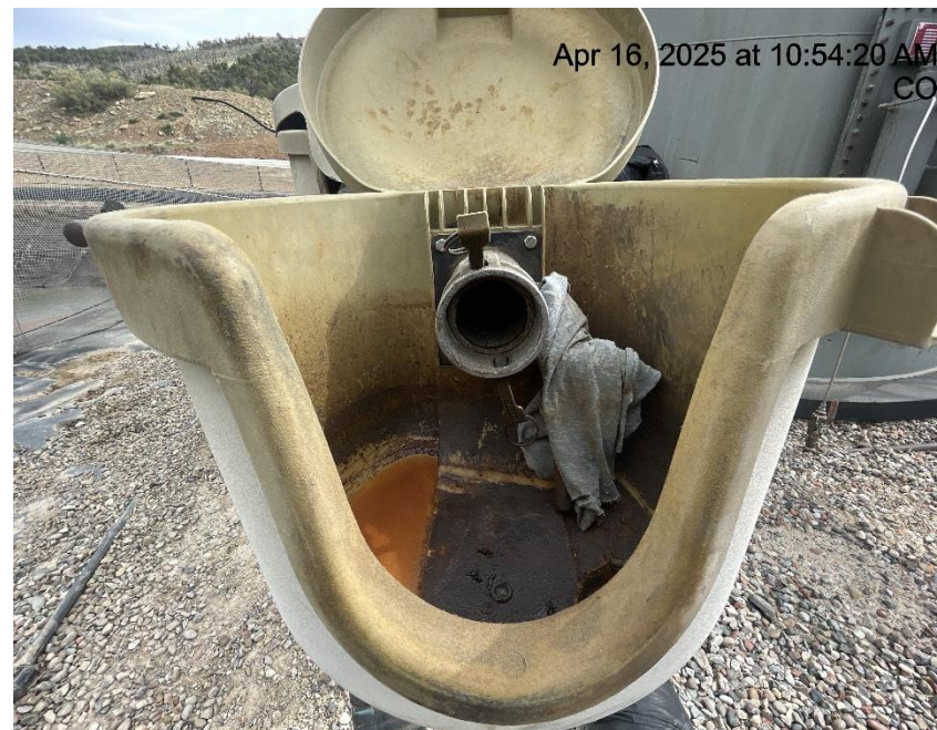
Photo # 1476 Open ended load line
