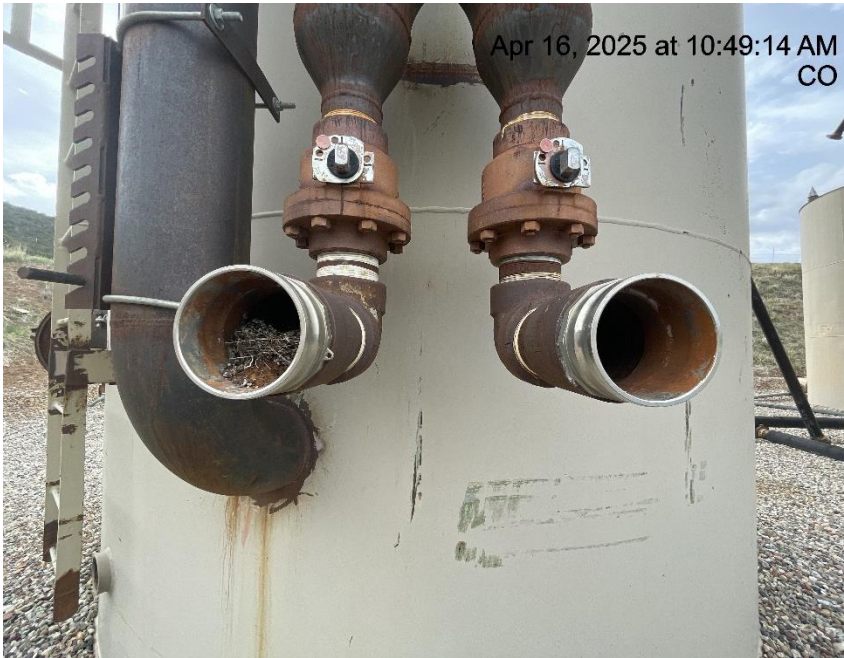
Photo # 1469 Open ended pipe/load lines on unused tank/wildlife hazard/available for entry by wildlife
