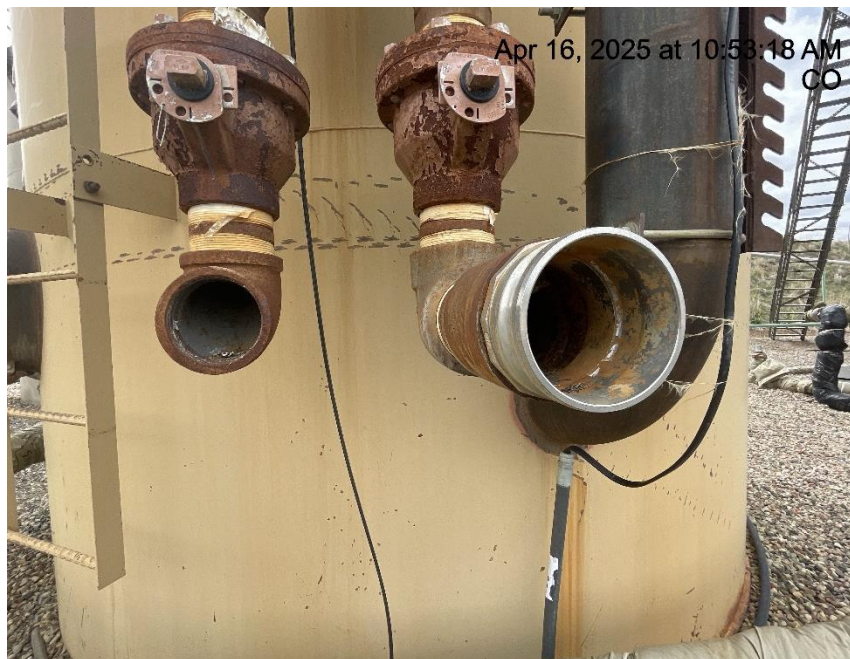
Photo # 1477 Open ended load lines
