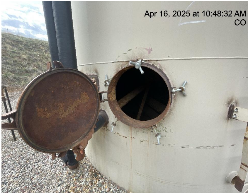
Photo # 1467 Open manway on unused tank/wildlife hazard/available for entry by wildlife
