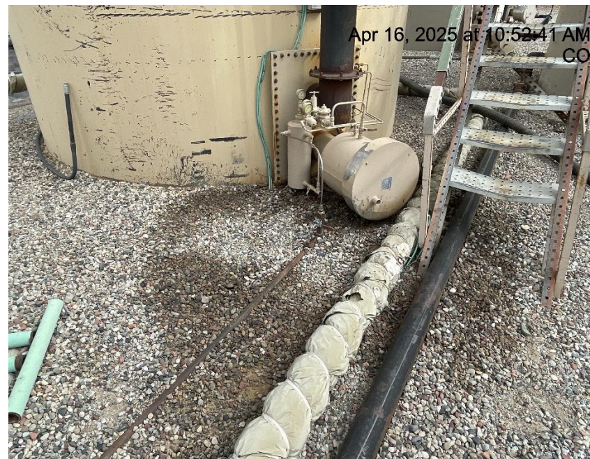
Photo # 1478 Staining in secondary containment
