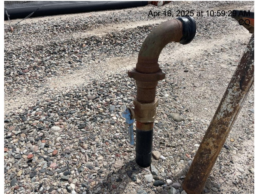
Photo # 1484 Unused riser line lacks lockout tagout (OOSLAT)
