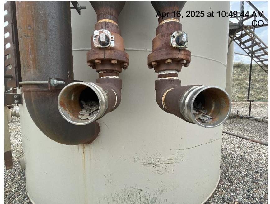
Photo # 1470 Open ended pipe/load lines on unused tank/wildlife hazard/available for entry by wildlife
