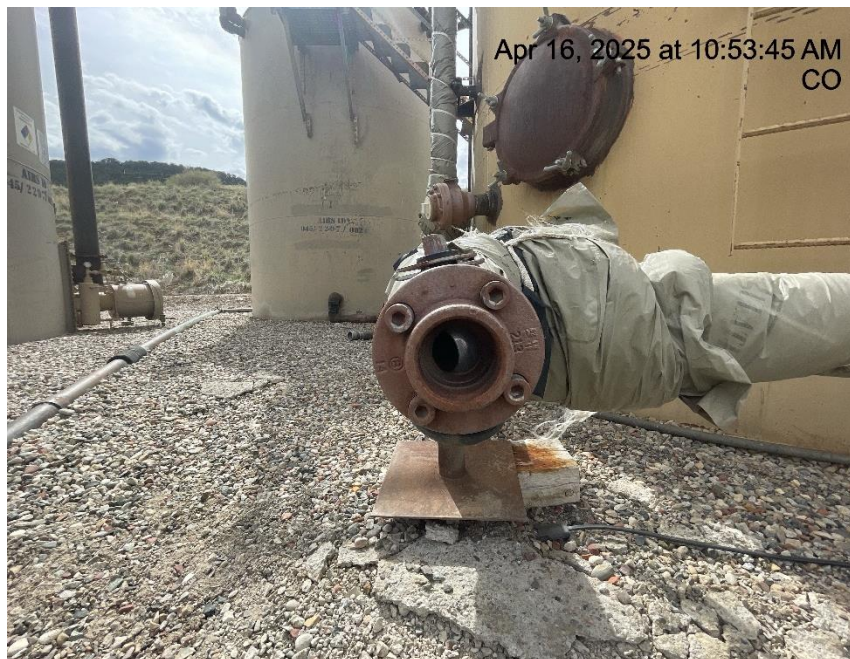
Photo # 1475 Open ended load line
