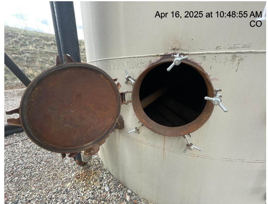
Photo # 1468 Open manway on unused tank/wildlife hazard/available for entry by wildlife
