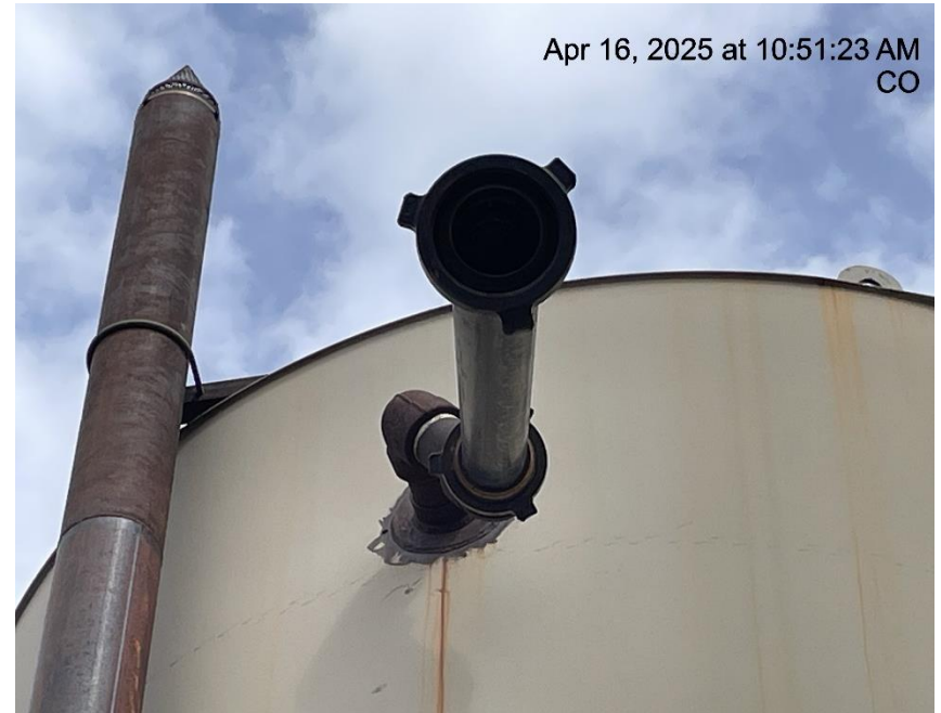
Photo # 1474 Open ended piping on unused tank/wildlife hazard/available for entry by wildlife
