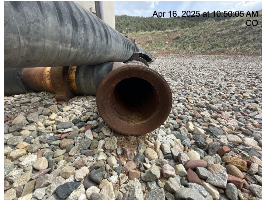
Photo # 1472 Open ended piping on unused tank/wildlife hazard/available for entry by wildlife
