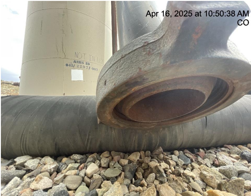
Photo # 1773 Open ended piping on unused tank/wildlife hazard/available for entry by wildlife
