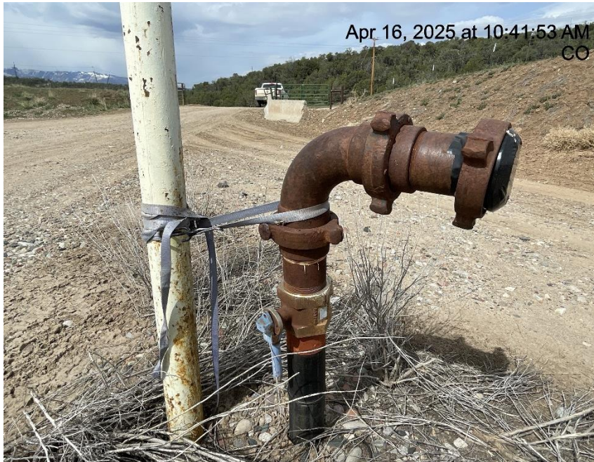
Photo # 1483 Unused riser line lacks lockout tagout (OOSLAT)
