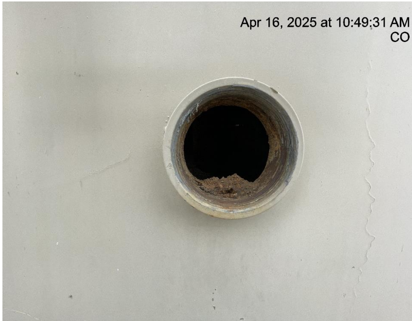
Photo # 1471 Open ended port on unused tank/wildlife hazard/available for entry by wildlife
