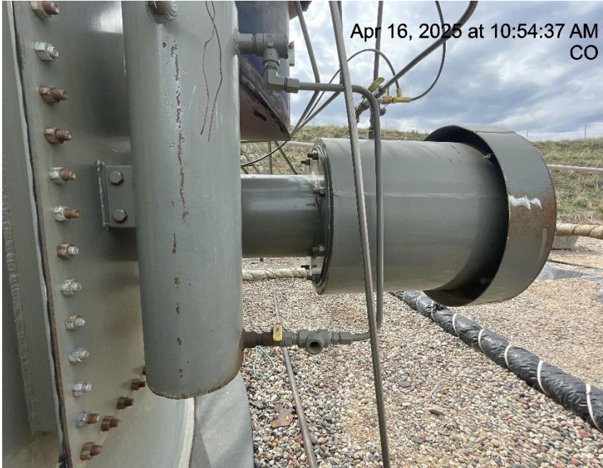
Photo # 1485 PRV vent line does not comply with CECMC pressure safety device rules
