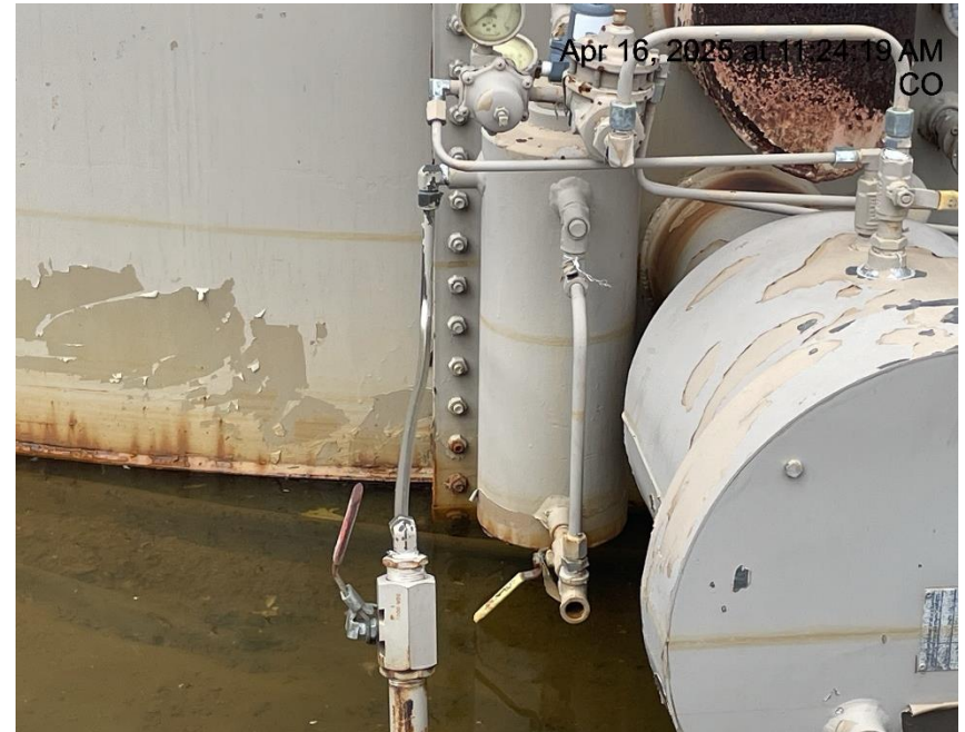
Photo # 1639 PRV vent line does not comply with CECMC pressure safety rules or general safety rules
