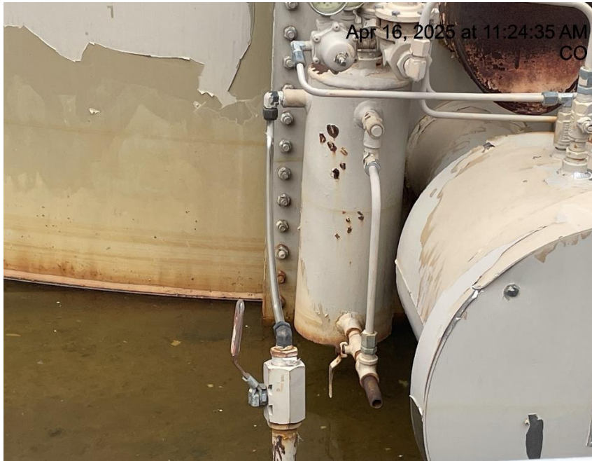
Photo # 1640 PRV vent line does not comply with CECMC pressure safety rules or general safety rules
