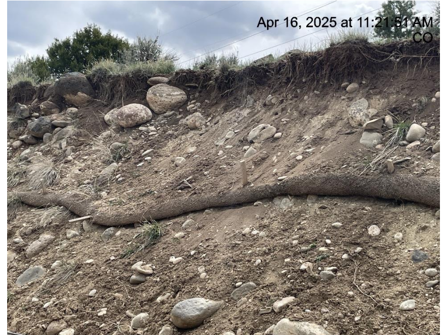
Photo # 1643 Lack of stabilization on cut slope/BMP's need maintenance
