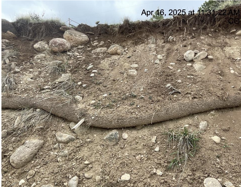
Photo # 1646 Lack of stabilization on cut slope/BMP's need maintenance
