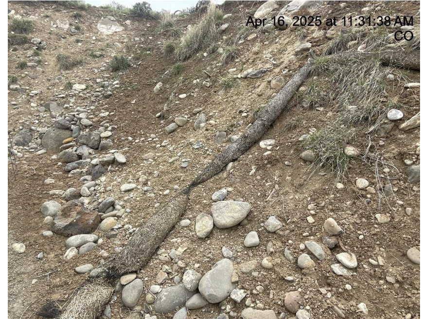
Photo # 1645 Lack of stabilization on cut slope/BMP's need maintenance
