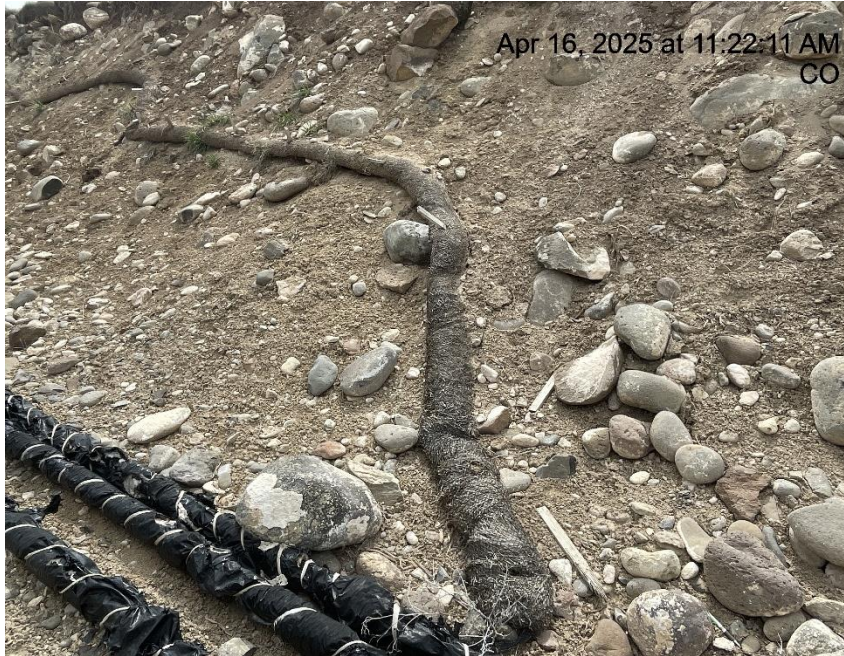
Photo # 1642 Lack of stabilization on cut slope/BMP's need maintenance
