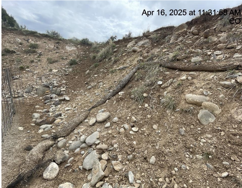
Photo # 1644 Lack of stabilization on cut slope/BMP's need maintenance
