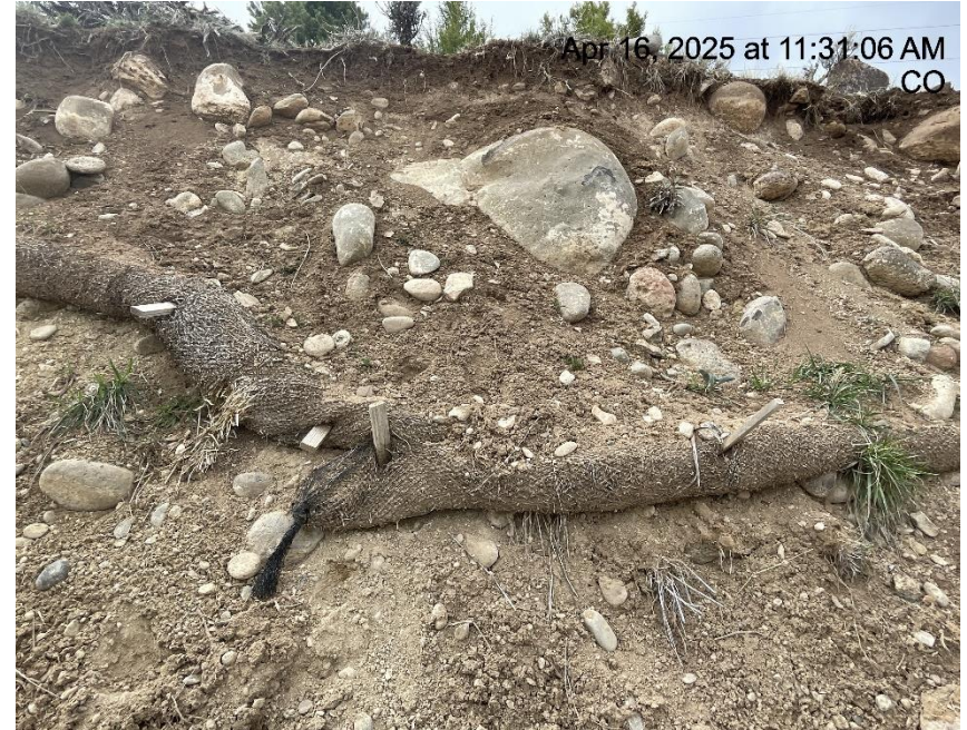
Photo # 1647 Lack of stabilization on cut slope/BMP's need maintenance
