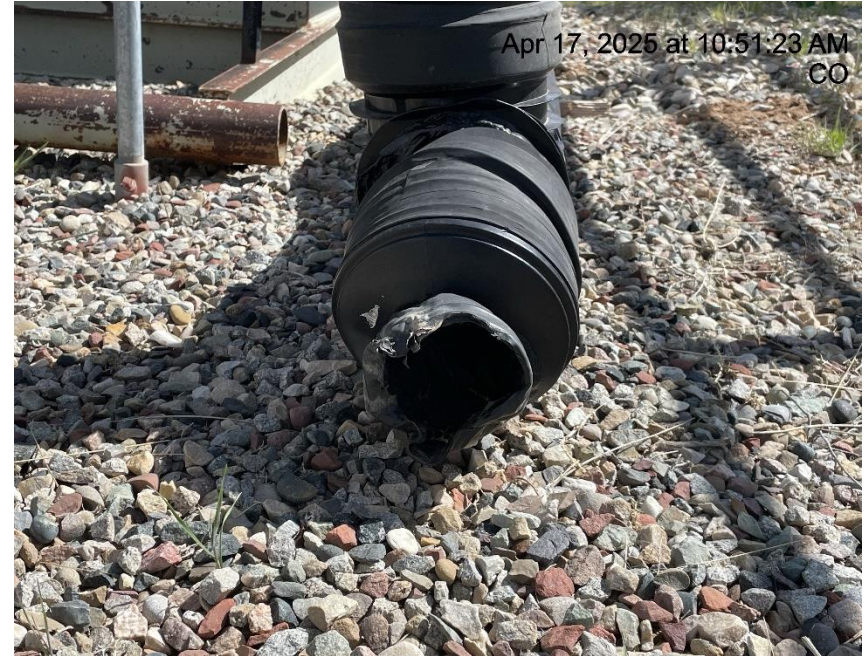
Photo # 2391 Flowline heating insulation open ended /wildlife hazard/available for entry by wildlife
