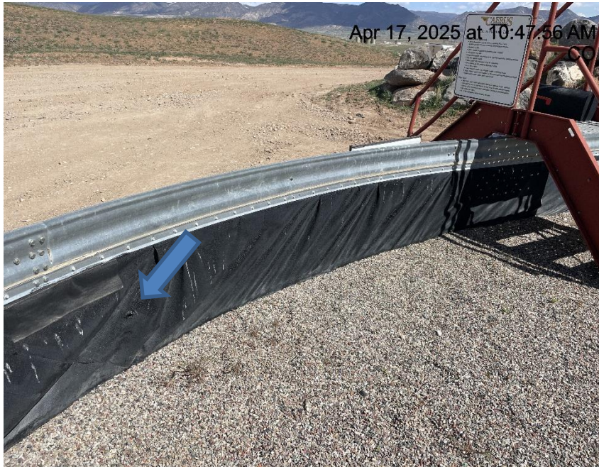
Photo # 2382 Hole in liner/liner needs maintenance
