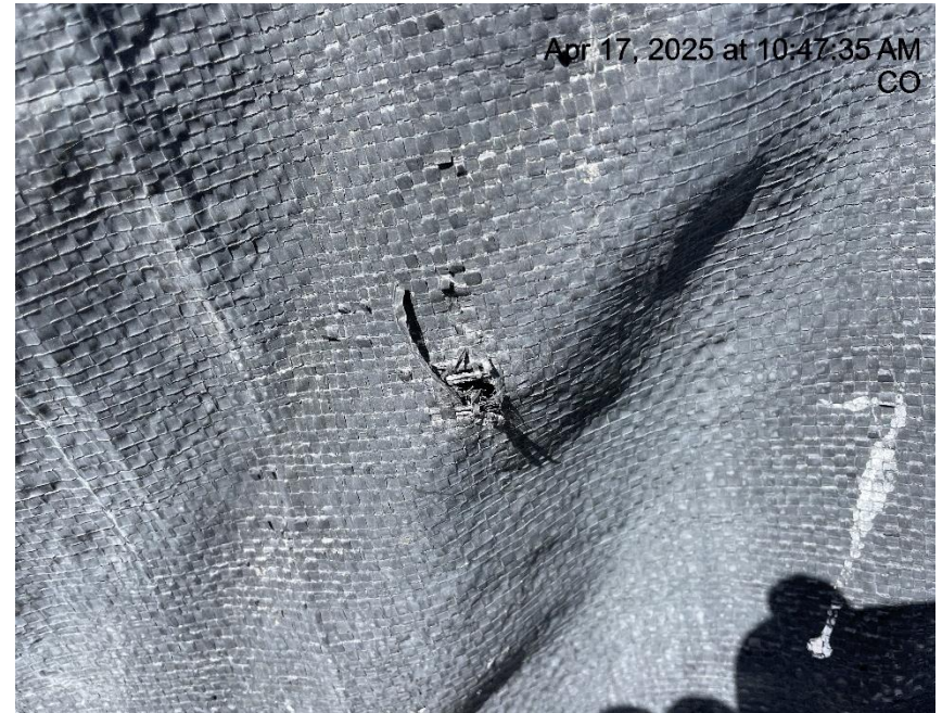
Photo # 2381 Hole in liner/liner needs maintenance
