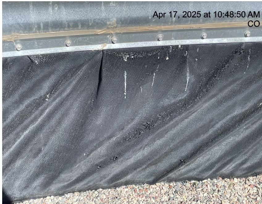
Photo # 2384 Holes in liner/liner needs maintenance & liner showing signs of deterioration
