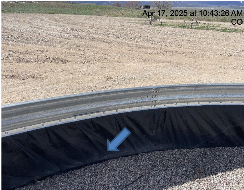
Photo # 2376 Hole in liner/liner needs maintenance
