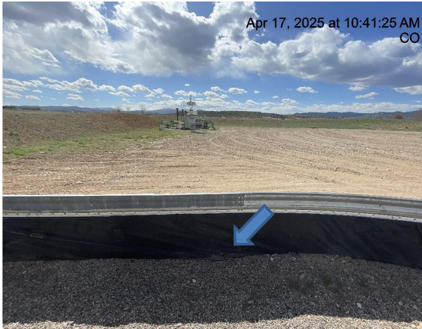
Photo # 2370 Hole in liner/liner needs maintenance
