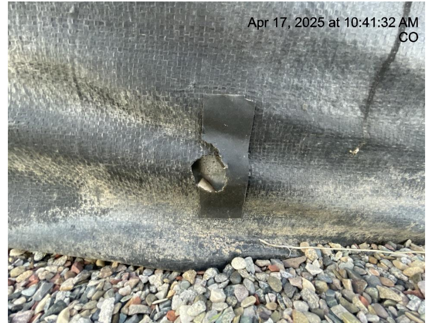
Photo # 2371 Hole in liner/liner needs maintenance
