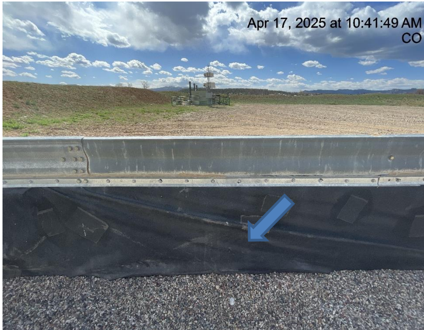
Photo # 2372 Hole in liner/liner needs maintenance
