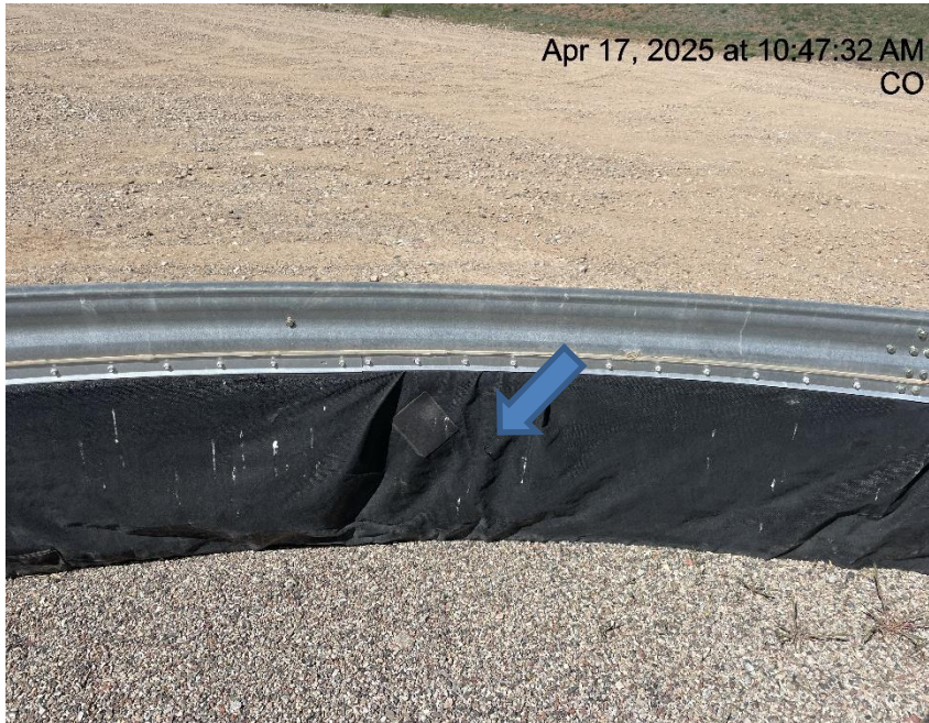
Photo # 2380 Hole in liner/liner needs maintenance
