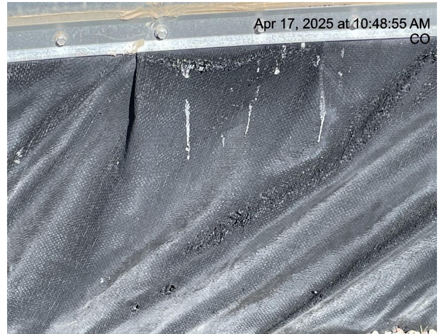
Photo # 2385 Holes in liner/liner needs maintenance & liner showing signs of deterioration
