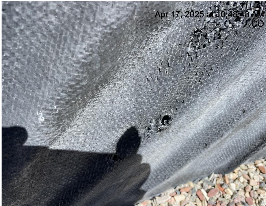
Photo # 2386 Hole in liner/liner needs maintenance & liner showing signs of deterioration
