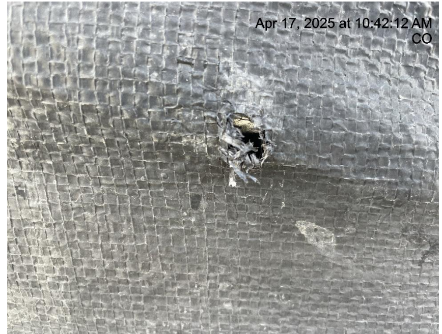
Photo # 2373 Hole in liner/liner needs maintenance
