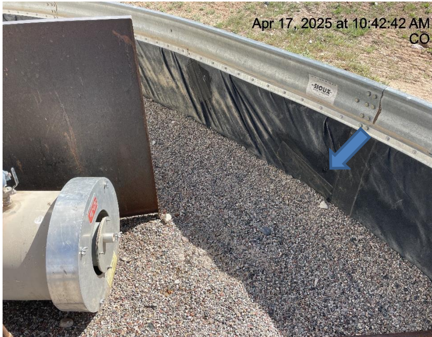
Photo # 2374 Hole in liner/liner needs maintenance
