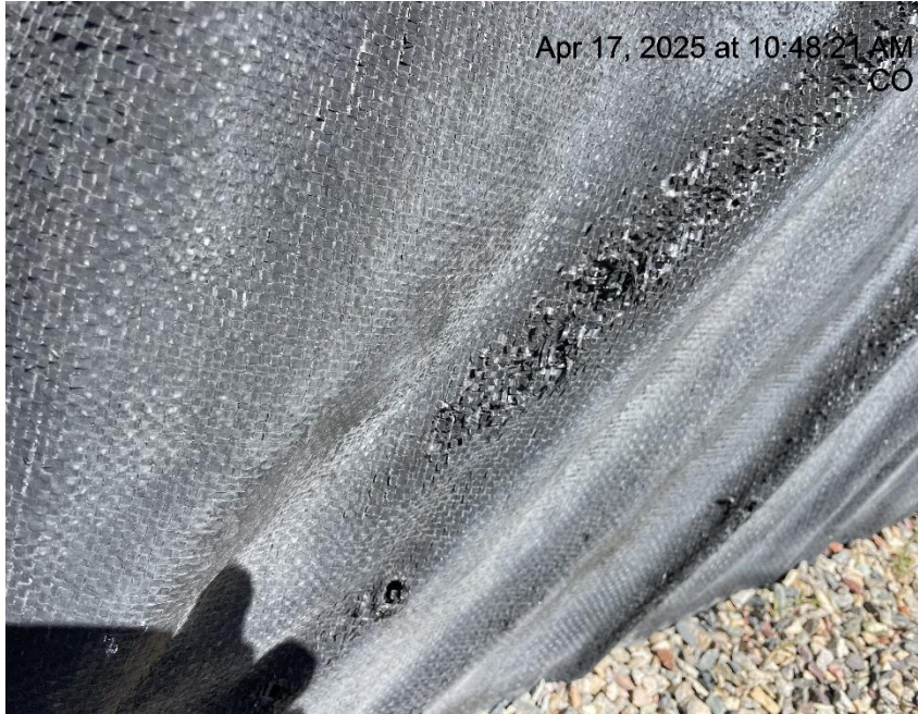
Photo # 2390 Hole in liner/liner needs maintenance & liner showing signs of deterioration
