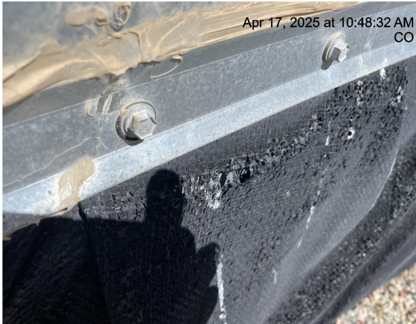
Photo # 2388 Hole in liner/liner needs maintenance & liner showing signs of deterioration
