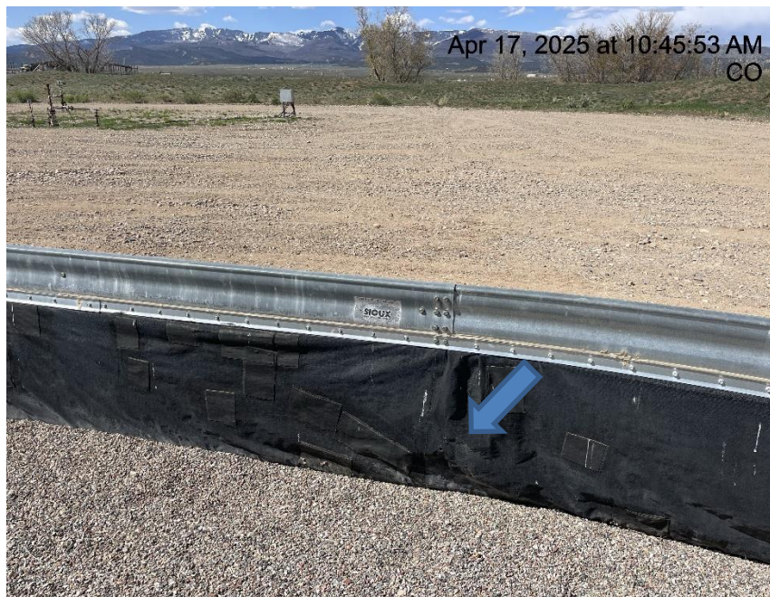
Photo # 2378 Holes in liner/liner needs maintenance
