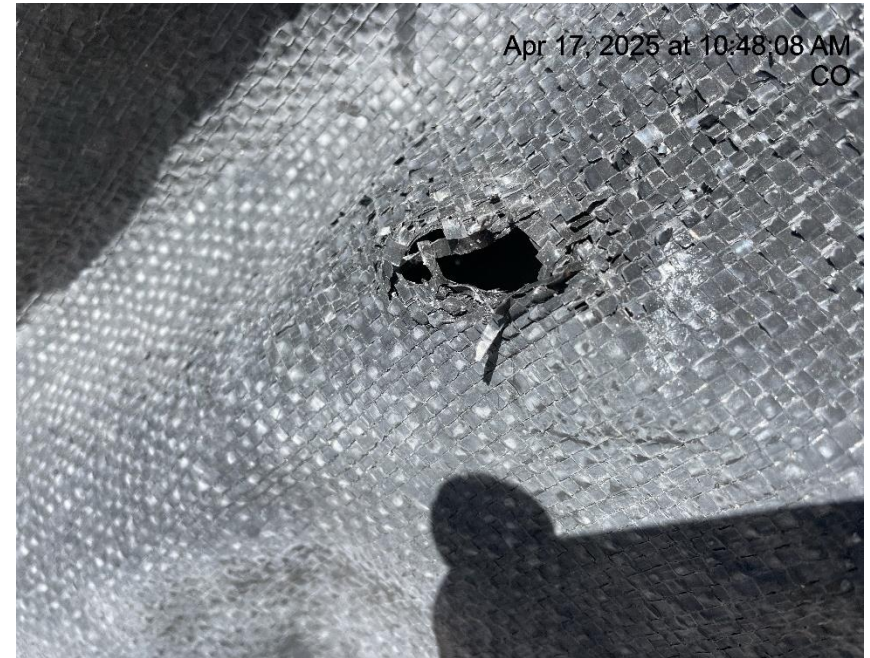
Photo # 2383 Hole in liner/liner needs maintenance & liner showing signs of deterioration
