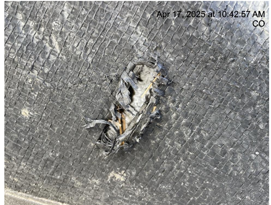
Photo # 2375 Hole in liner/liner needs maintenance
