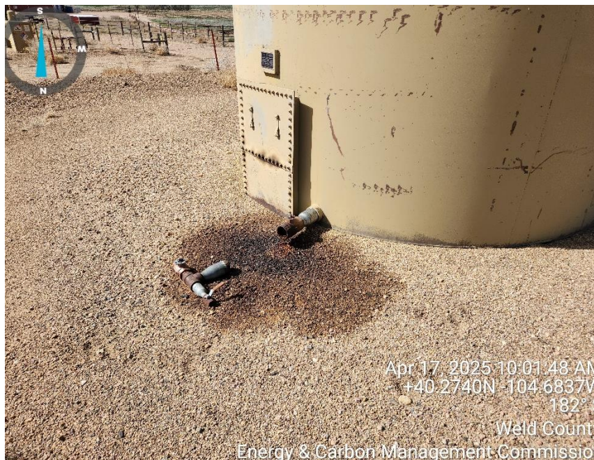
Photo 3 stained soil crude tank drain
