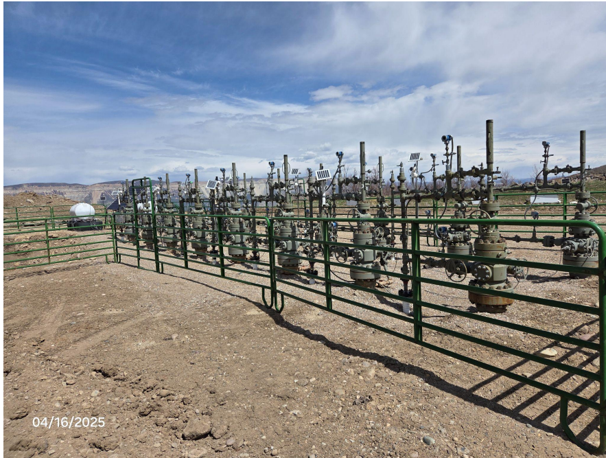
Photo 6: Photos examples showing signage missing from wells.
