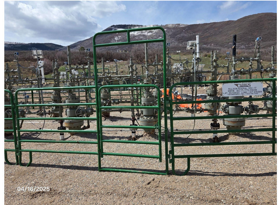
Photo 6: Photos examples showing signage missing from wells.
