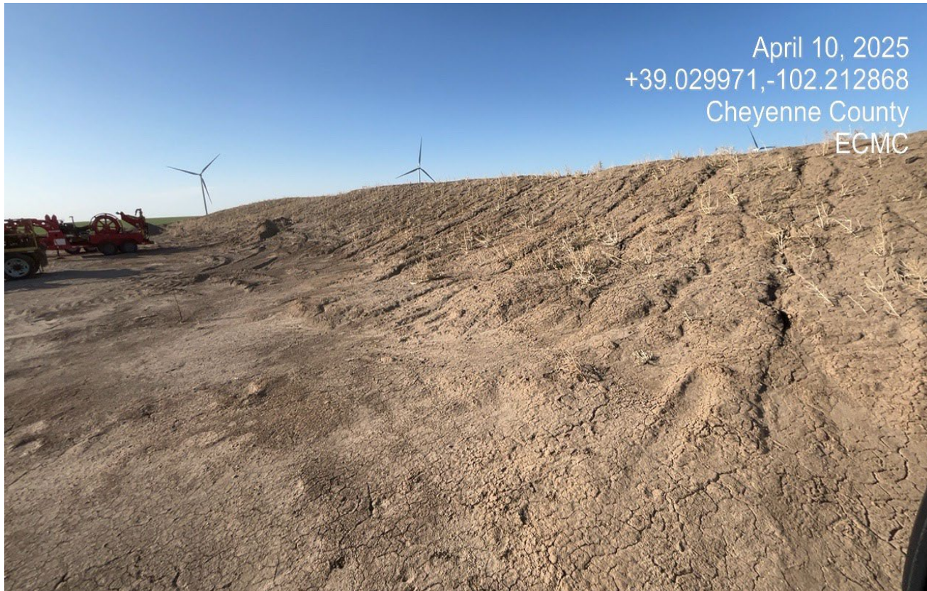
Photo 8. Facing toward the topsoil pile which is not stabilized and has not been replaced.
