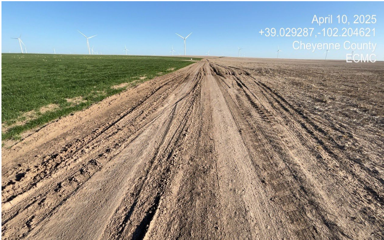
Photo 1. Facing north along the main road leading to the location. There is vehicle rutting and signs of vehicles going outside of the road causing unnecessary disturbance.
