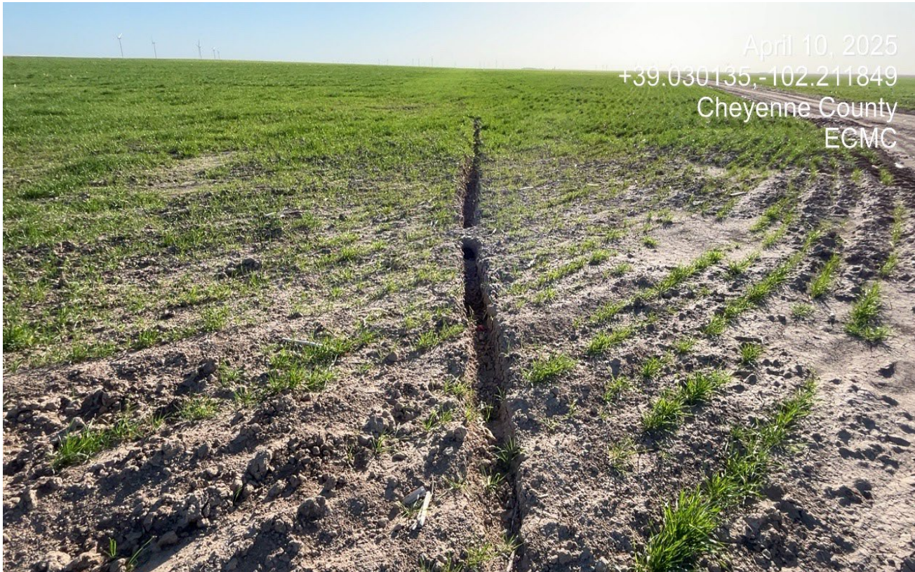
Photo 6. There is subsidence along the flowline.
