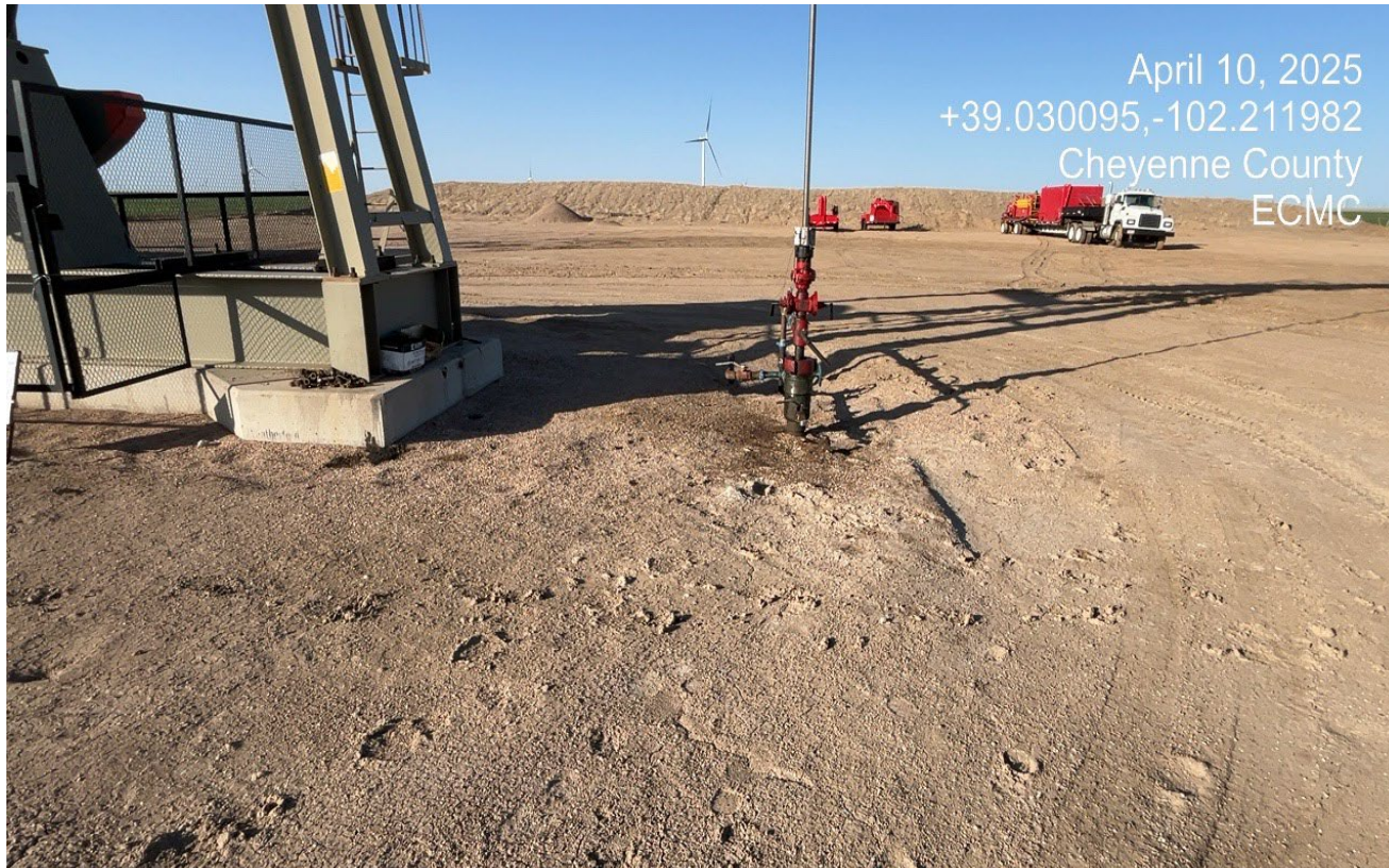
Photo 4. There is stained soils at the wellhead.
