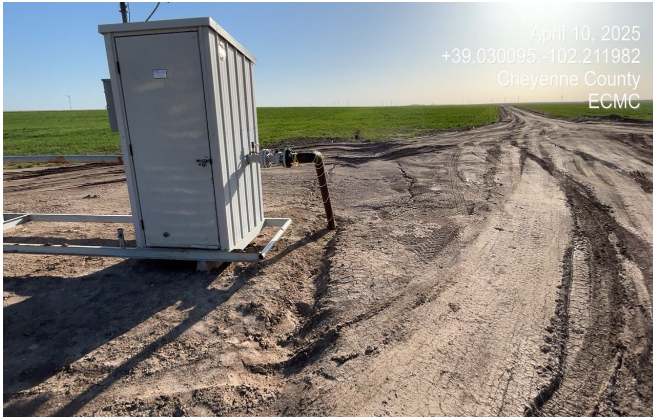
Photo 5. There is subsidence at the meter shed along the flowline.
