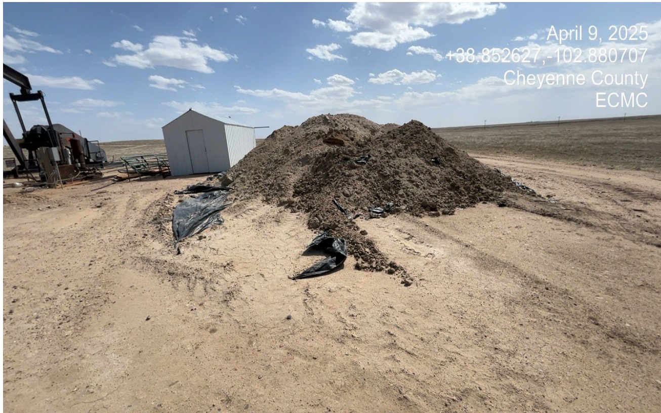
Photo 2. The impacted soils are not being stored with containment and have spread off of the plastic liner.
