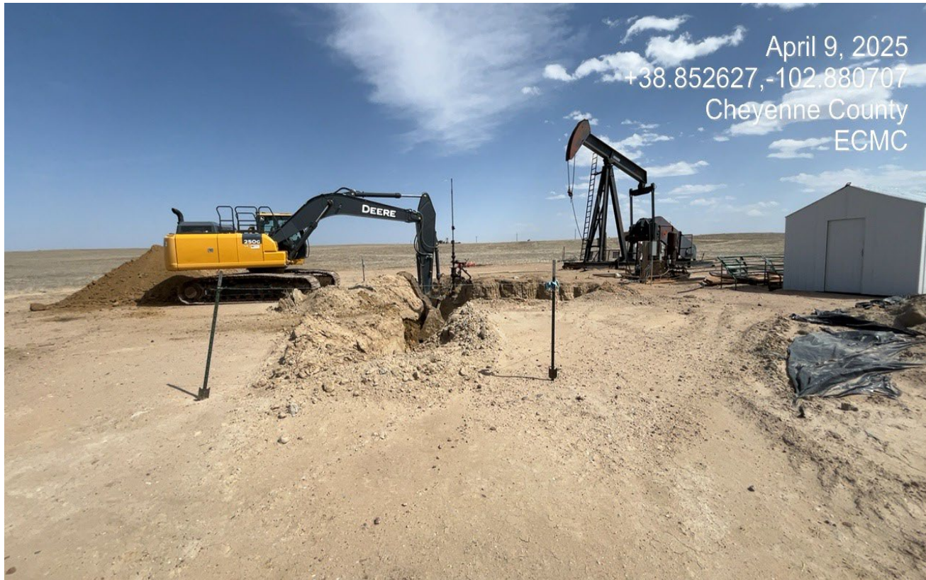
Photo 3. There was excavation occurring at the wellhead during the inspection. The excavated area must be fenced off to prevent wildlife or livestock entry.
