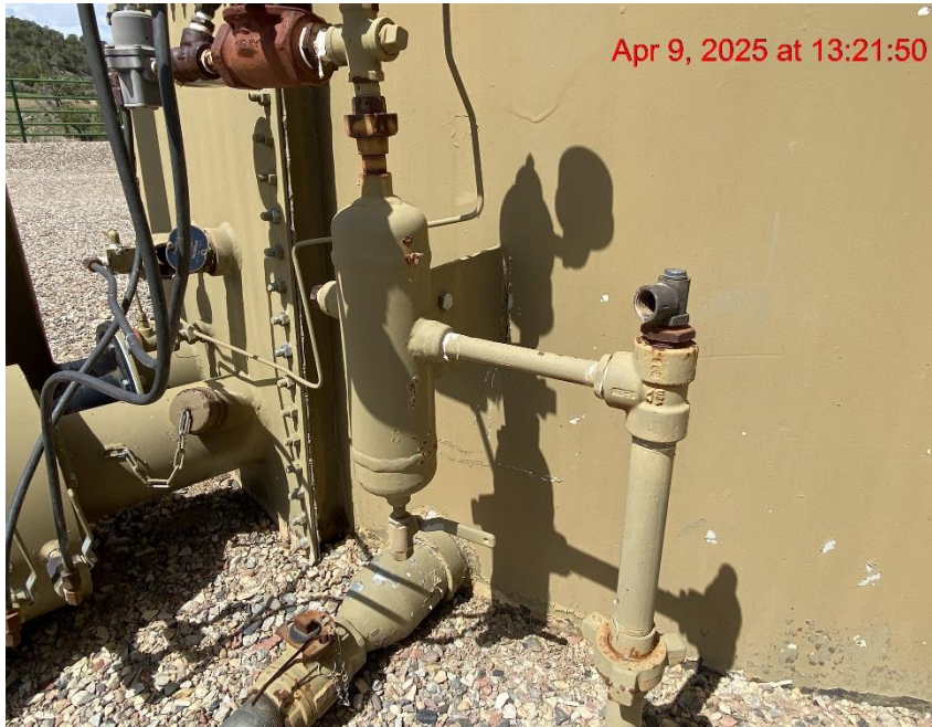
PRV Terminates in Unsafe Manner – Photo #08068
