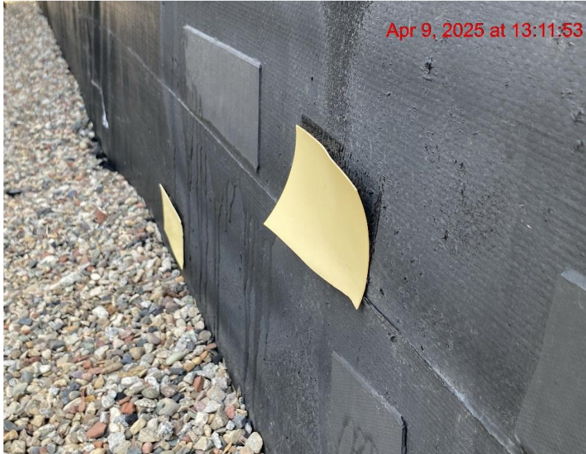
Berm Liner Patch is Peeling – Photo #08053
