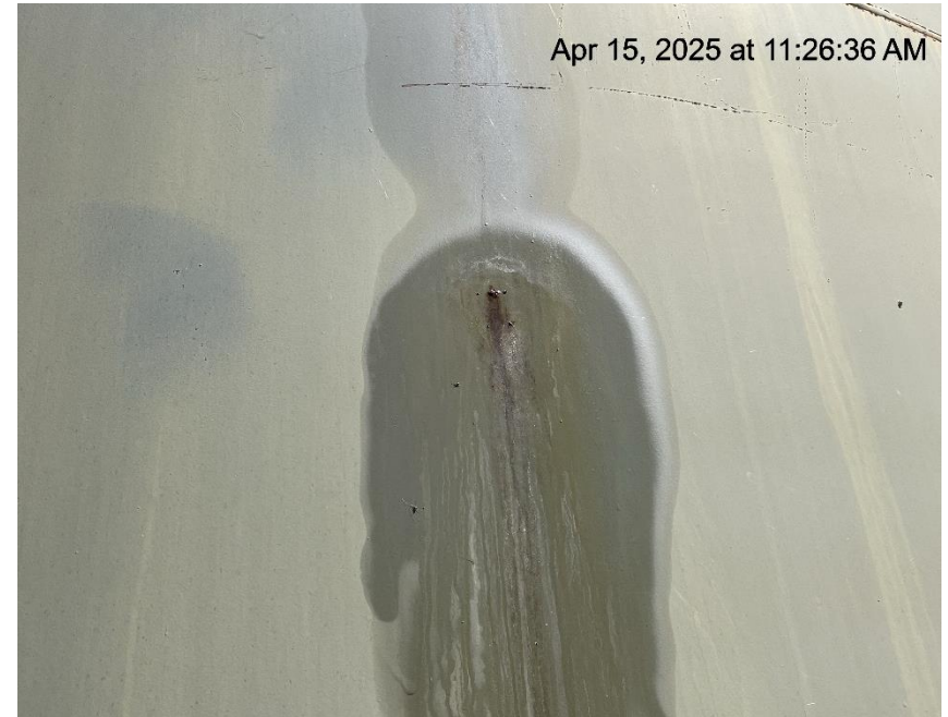
Photo # 1282 Possible tank failure - Suspected leak on production tank/tank appears to lack integrity
