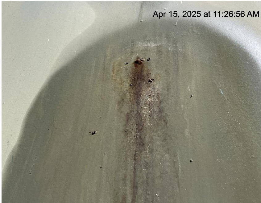
Photo # 1283 Possible tank failure - Suspected leak on production tank/tank appears to lack integrity
