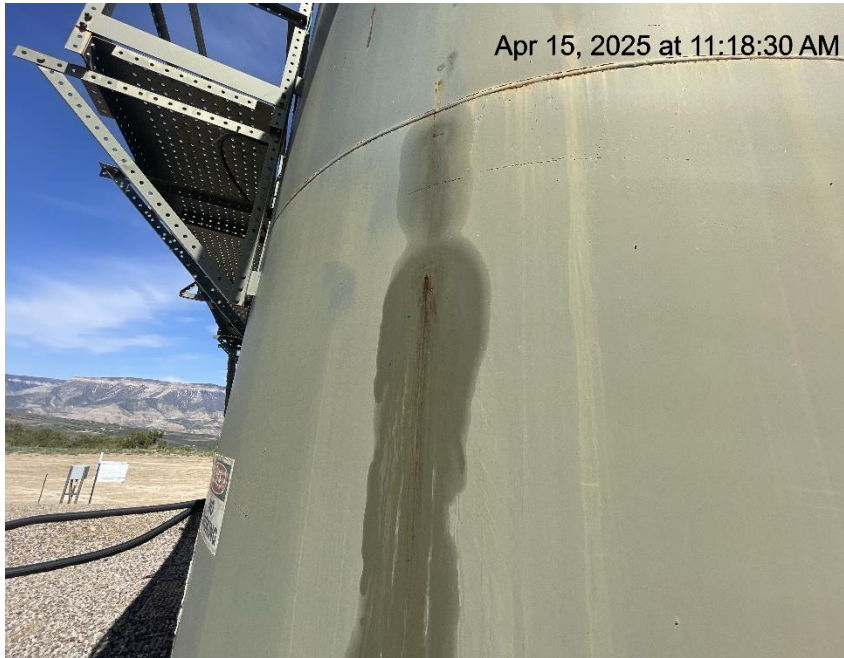
Photo # 1281 Possible tank failure - Suspected leak on production tank/tank appears to lack integrity
