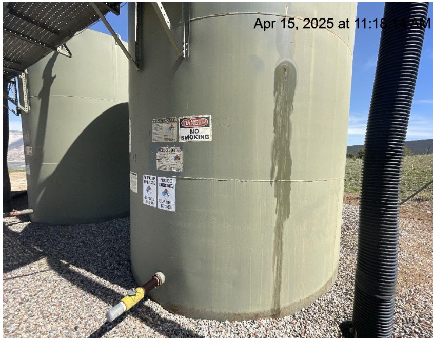
Photo # 1279 Possible tank failure - Suspected leak on production tank/tank appears to lack integrity
