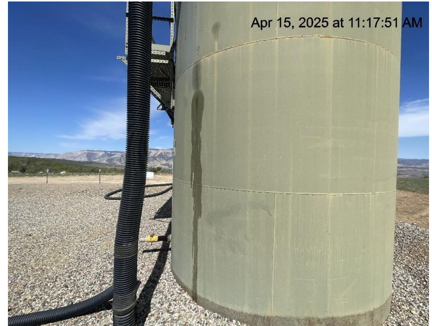
Photo # 1280 Possible tank failure - Suspected leak on production tank/tank appears to lack integrity
