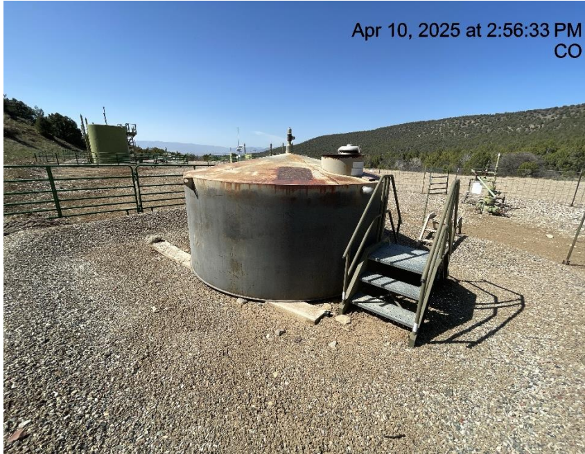
Photo # 625 Tank is disconnected & not in use/unused equipment
