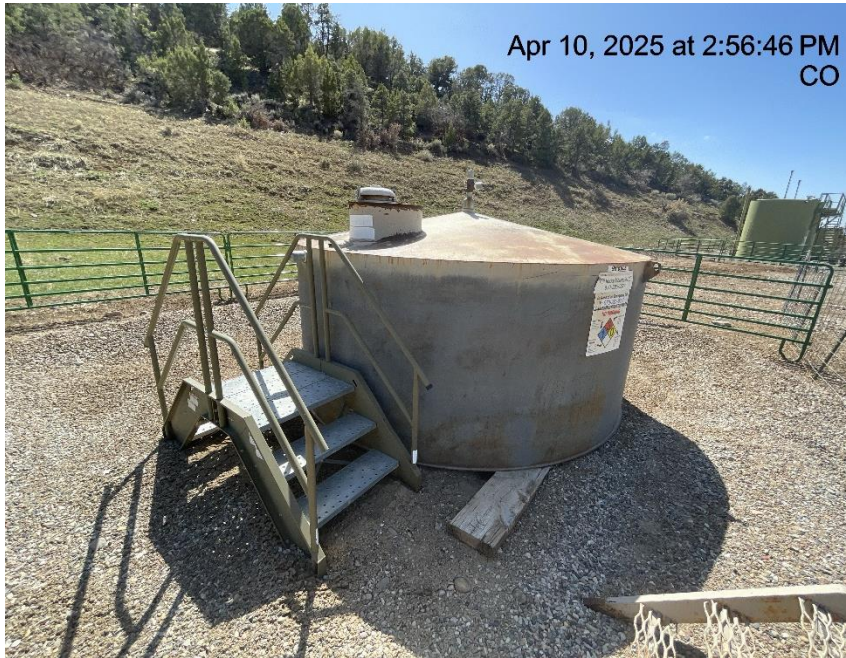
Photo # 623 Tank is disconnected & not in use/unused equipment
