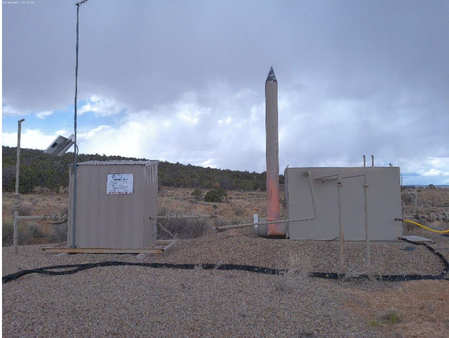
Separator and Meter housing.
