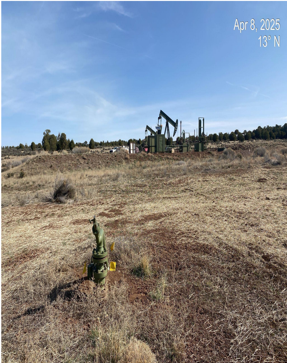
Photo 4. Gas line riser that remains in the northwest corner of the project area.
