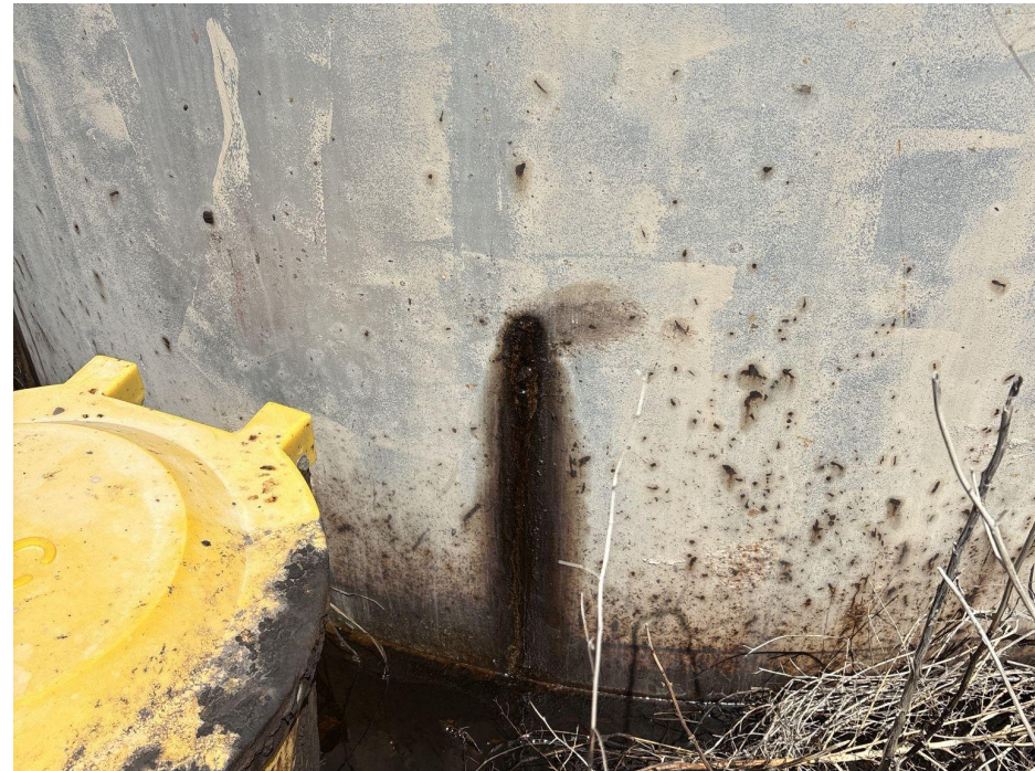
Photo 6. Looking at the west side of southern tank. Fluid appeared wet. Approximately 2ft above ground level.
