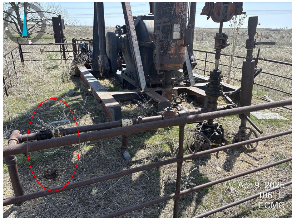
Photo 10. Pumpjack. Leaking fitting and stained soil beneath it (red circle).
