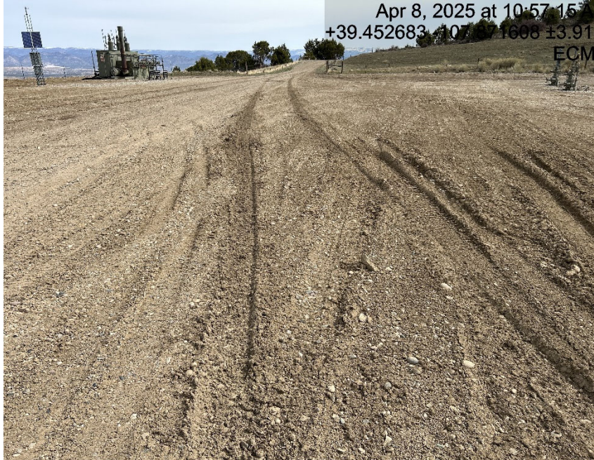
Lack of stabilization/compaction/tracking controls
