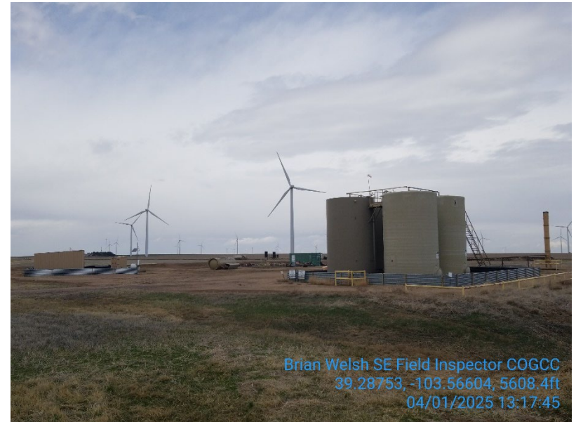
2. Tank battery and production equipment
