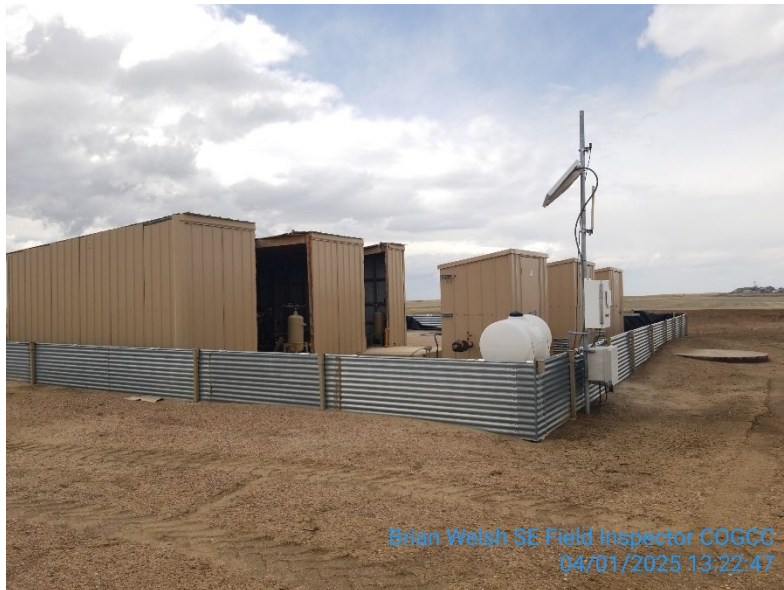
3. Meter shed and treater house. Treaters have been removed
