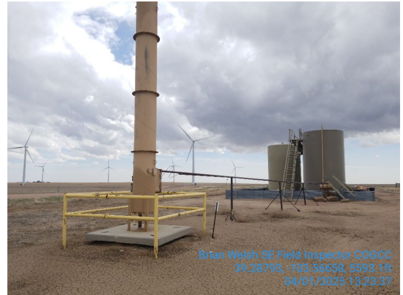
6. ECD (30") is on the north side of production tanks
