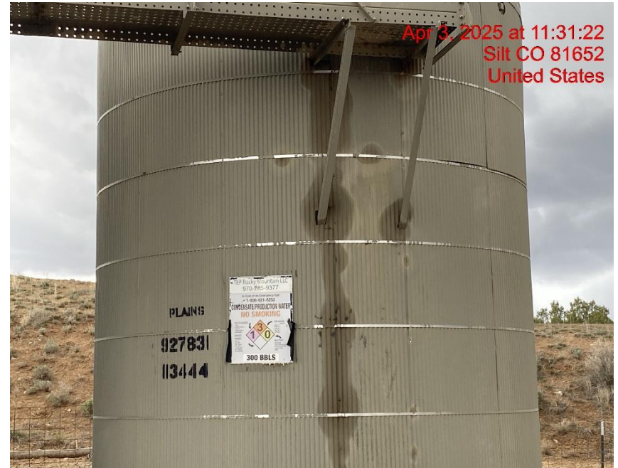
Staining on Tank – Photo #07914
