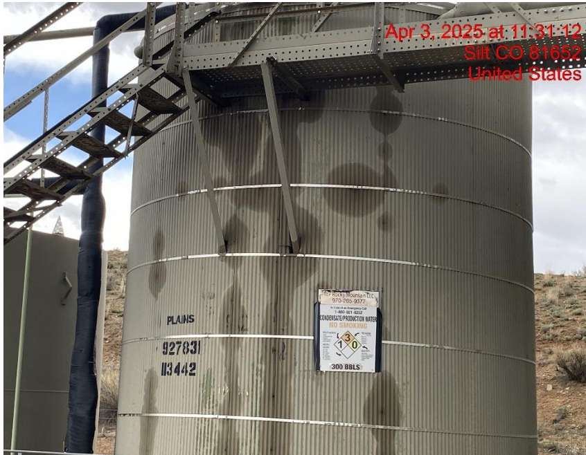
Staining on Tank – Photo #07913
