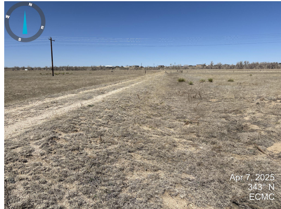
Photo 2. Access road is heavily contoured. It does not appear that the road was recontoured and graded to match surrounding landscape.
