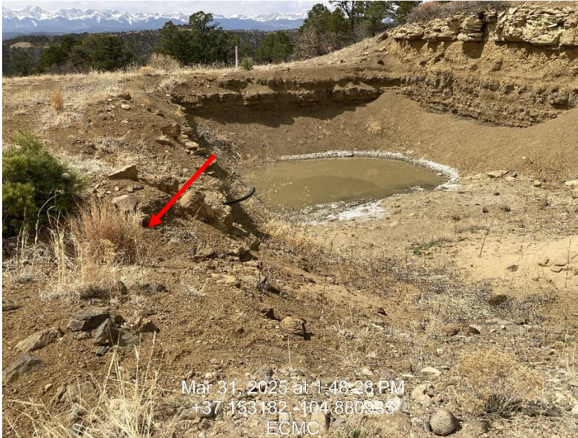
Photo 7 – Storm water entering pit
