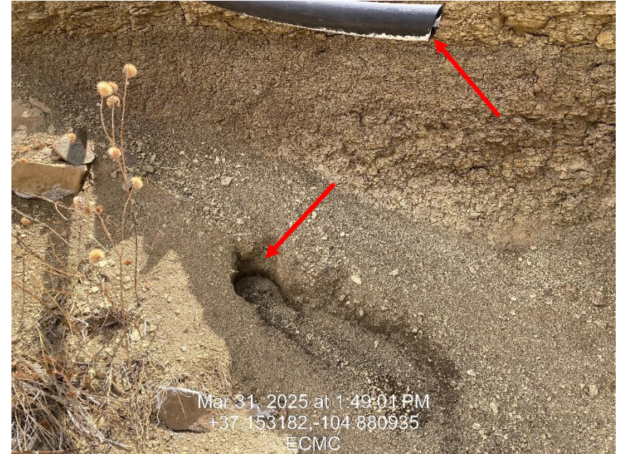
Photo 8 – Pit Dump Line, evidence of water flow from Dump Line into pit
