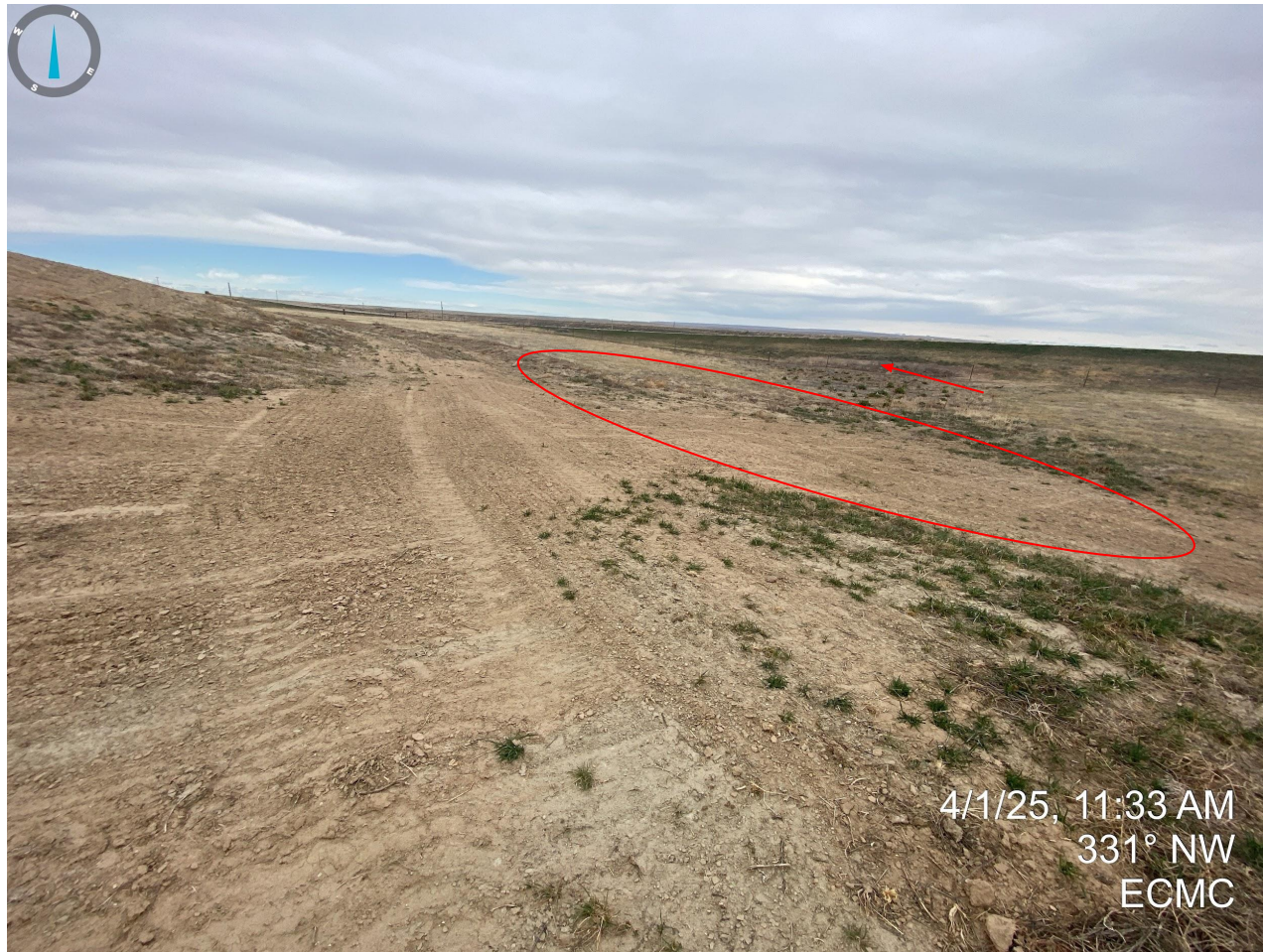
Photo 19. No apparent stormwater control measures observed on the north end of the location that would prevent sediment laden stormwater from exiting off location, into the culvert underneath CO HWY 14 (indicated by red arrow).
