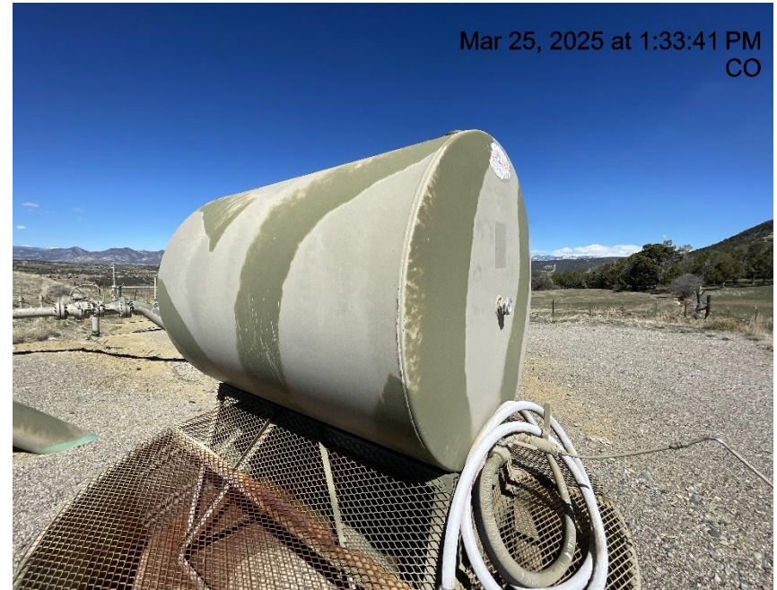
Photo # 7343 Methanol tank lacks required information
