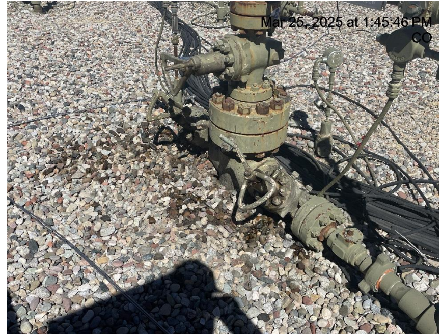
Photo # 7345 Staining near wellhead
