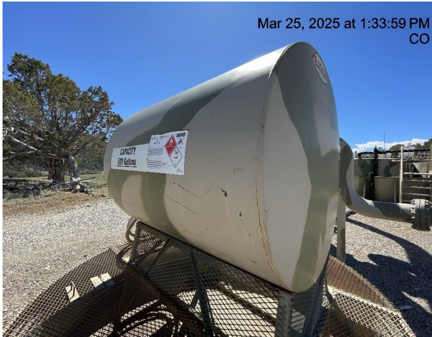
Photo # 7342 Methanol tank lacks required information
