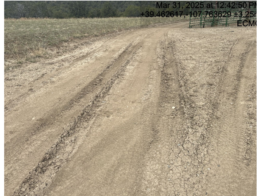
Lack of stabilization/ compaction
