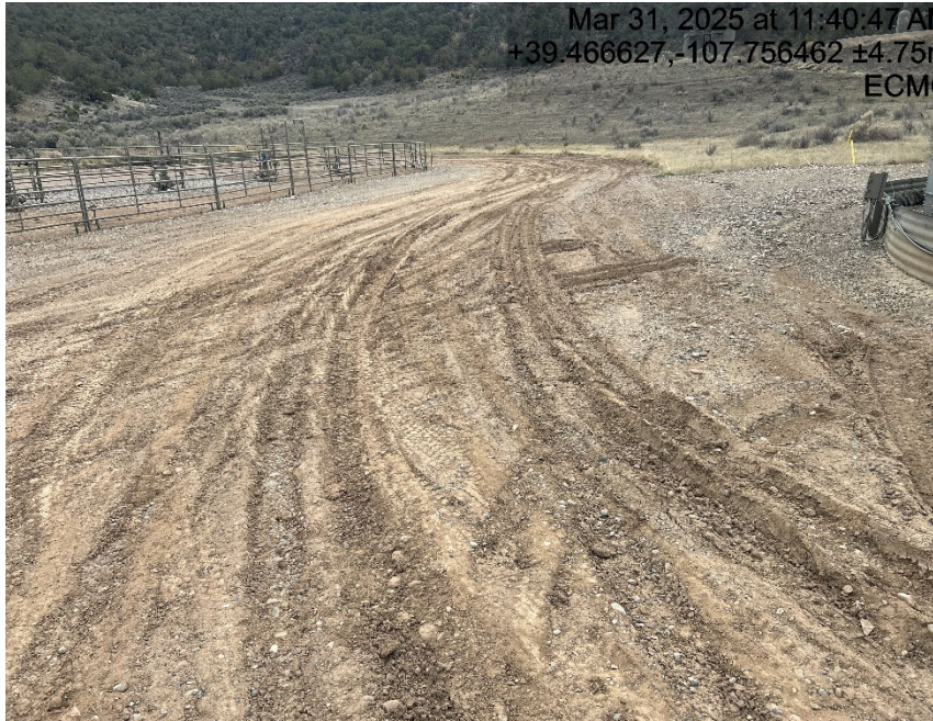
Some lack of stabilization/ compaction
