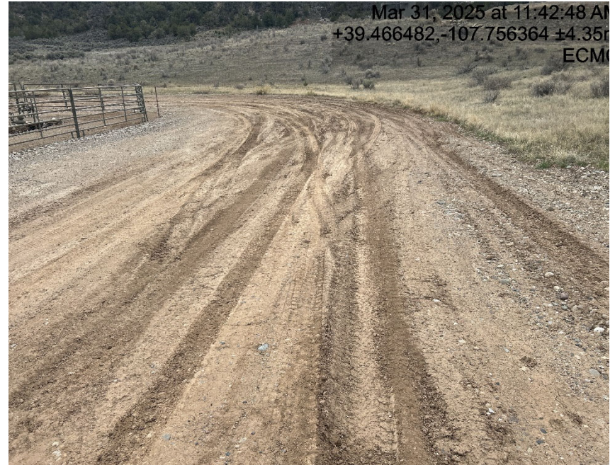
Some lack of stabilization/ compaction
