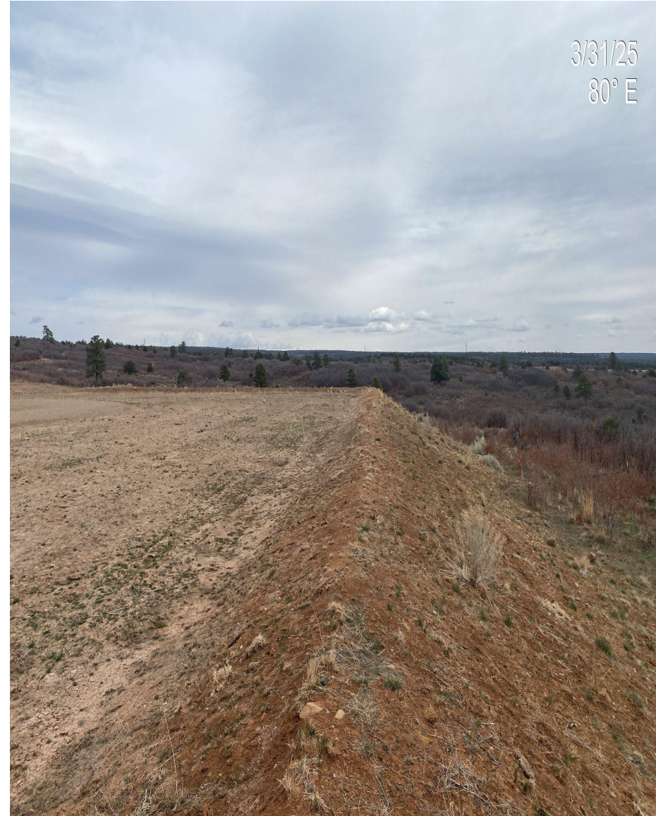
Photo 2. View of cut a fill slopes that have not been recontoured per 1003 standards.
