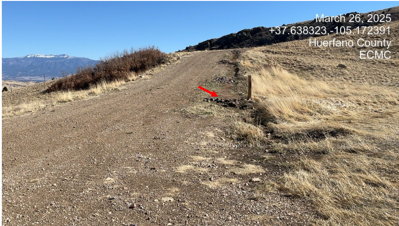
Photo 1. Facing northeast toward the access road. The rock check dams shown at red arrow are filled in with sediment and require maintenance.
