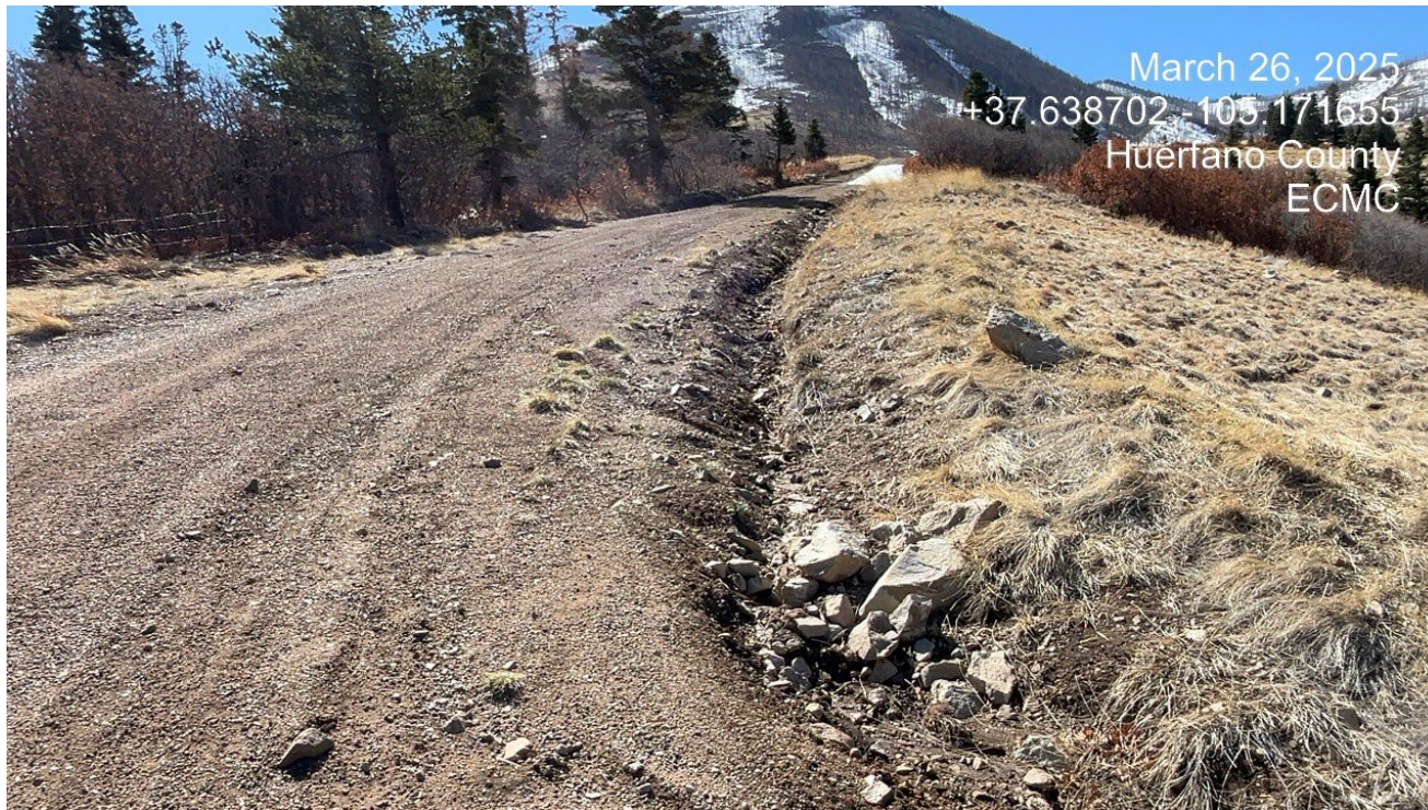
Photo 3. Facing southeast as the access road ascends to the location. There are insufficient BMP's to prevent erosion. Previous CA was not completed.
