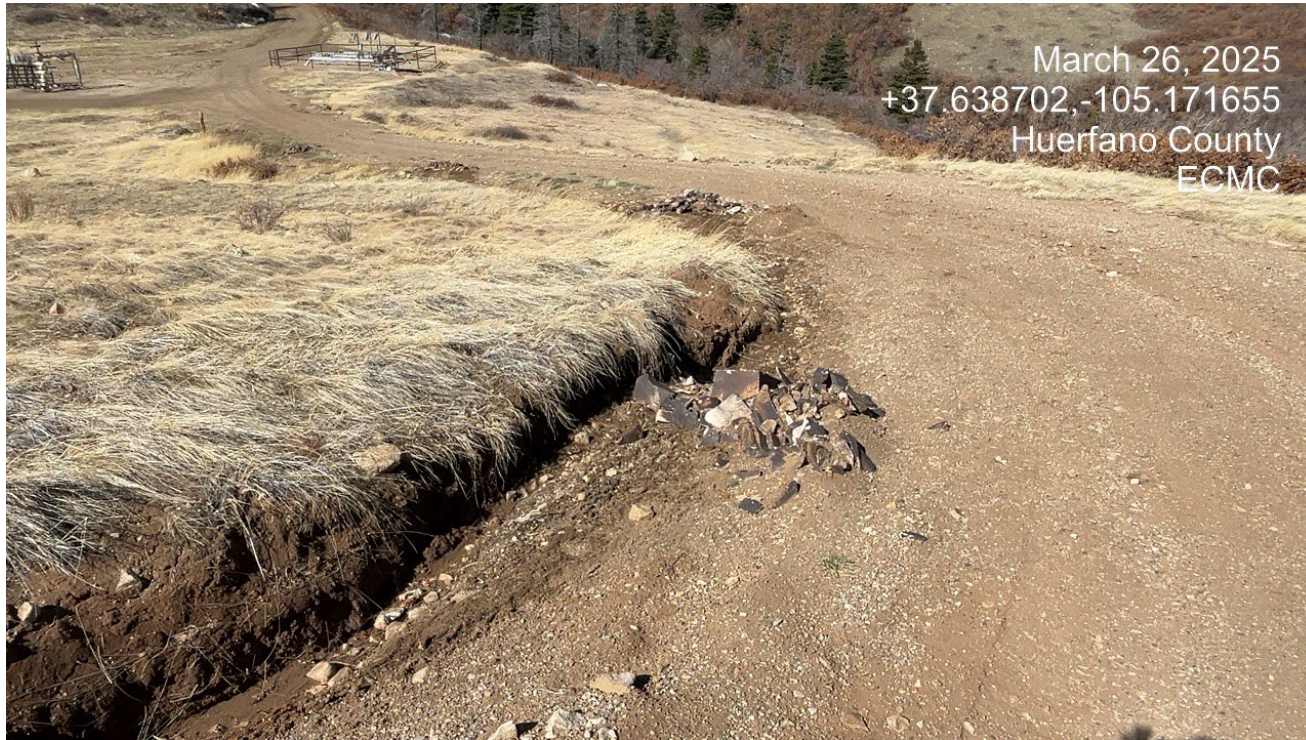
Photo 2. Facing back northwest along the access road. Theis check dam is in needof maintenance.
