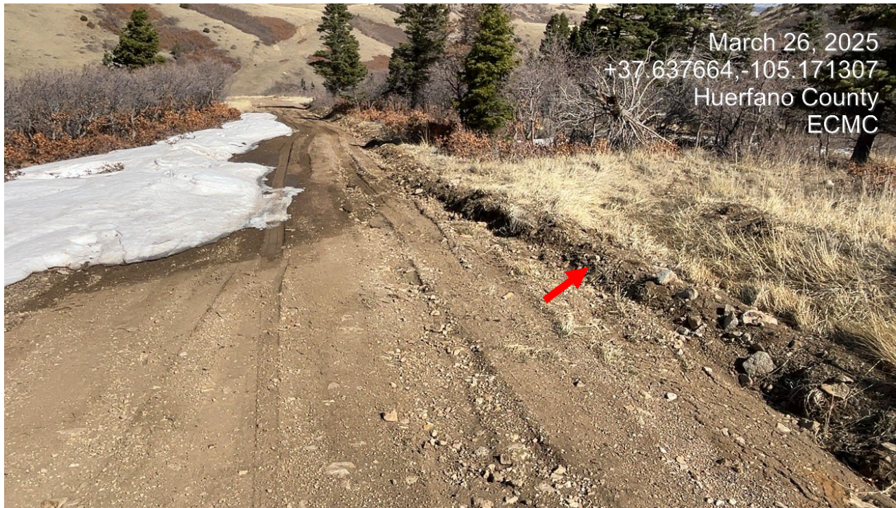
Photo 4. Facing back north the steep grade of access road. Stormwater is not being diverted off the road which is causing erosion of the road. Stormwater should be divert toward red arrow and into a sediment trap. A water bar would also help direct stormwater off the road.
