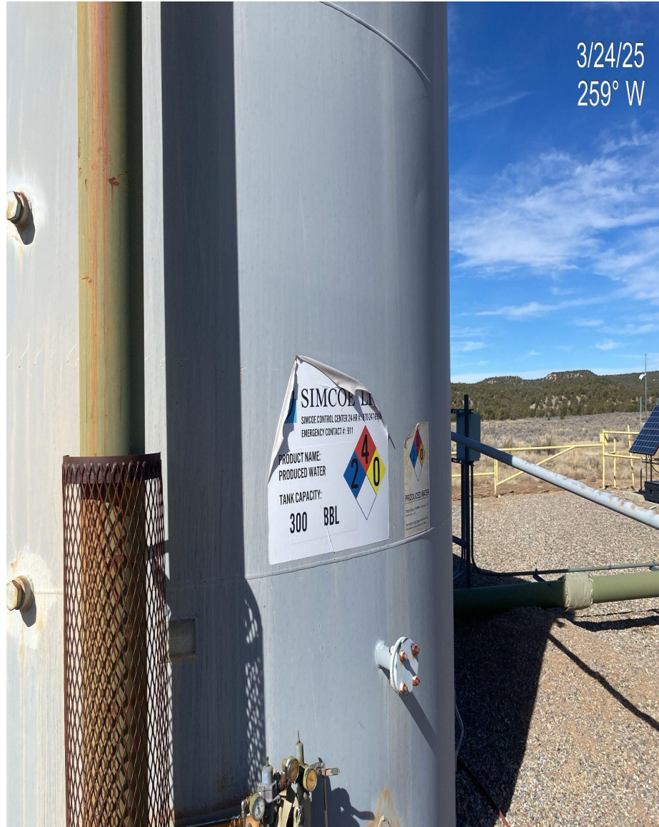
Photo 3. Produced water tank labels are starting to peel, future maintenance is advised.
