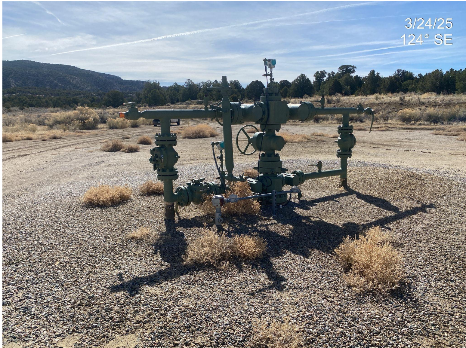
Photo 5. Weedy debris encroaching on wellhead.
