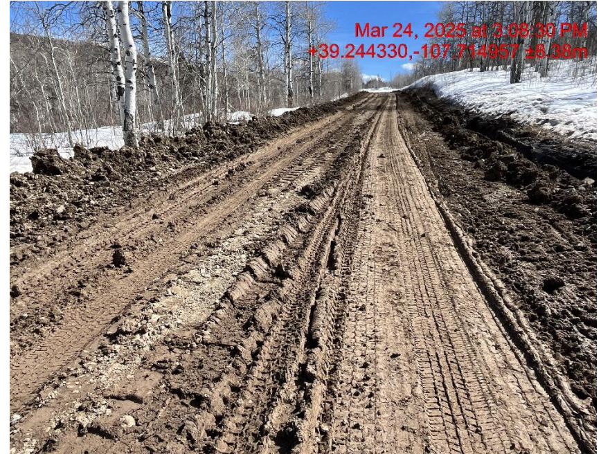
Photo # 6767 Vehicle tracking onto lease road/Insufficient tracking BMP's
