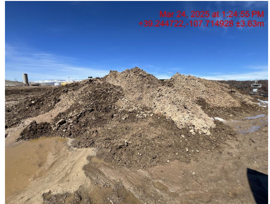
Photo # 6698 Stockpiled soils on location with no BMP's
