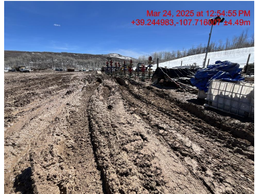
Photo # 6687 Lack of stabilization/compaction on location/insufficient tracking BMP's
