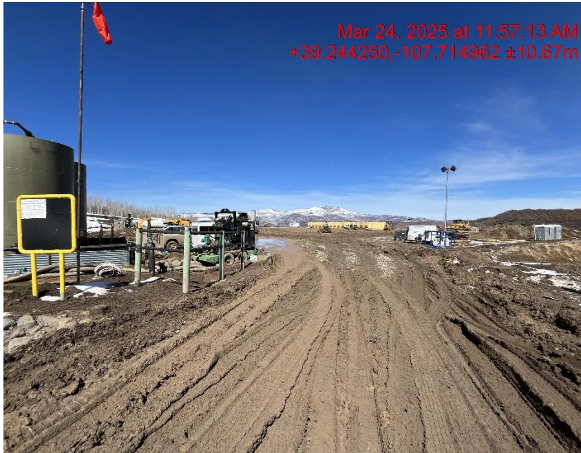
Photo # 6681 Entrance to location/Lack of stabilization/compaction/insufficient tracking BMP's
