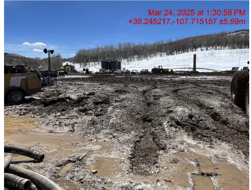
Photo # 6707 Lack of stabilization/compaction on location/insufficient tracking BMP's
