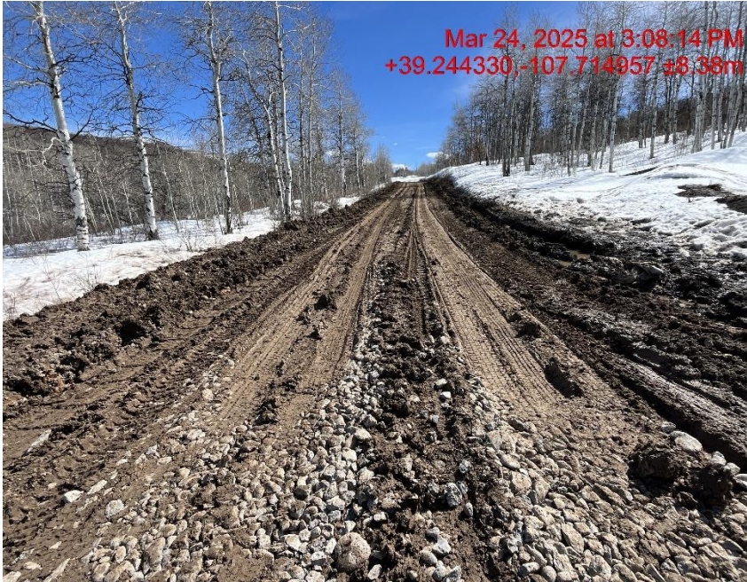
Photo # 6766 Vehicle tracking onto lease road/Insufficient tracking BMP's
