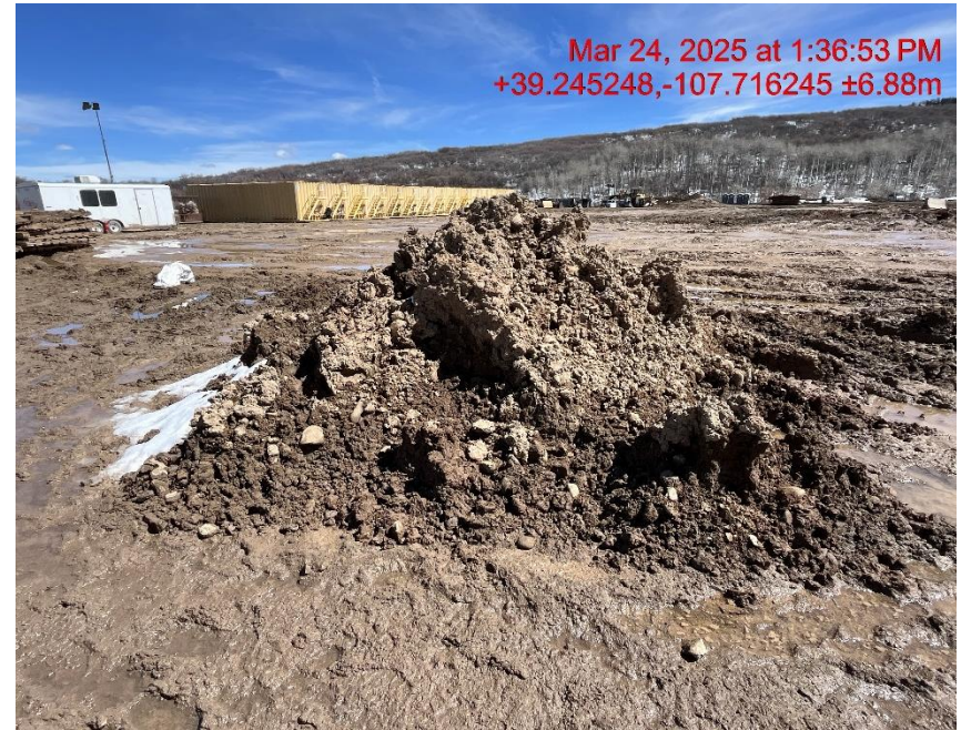
Photo # 6712 Stockpiled soils on location with no BMP's
