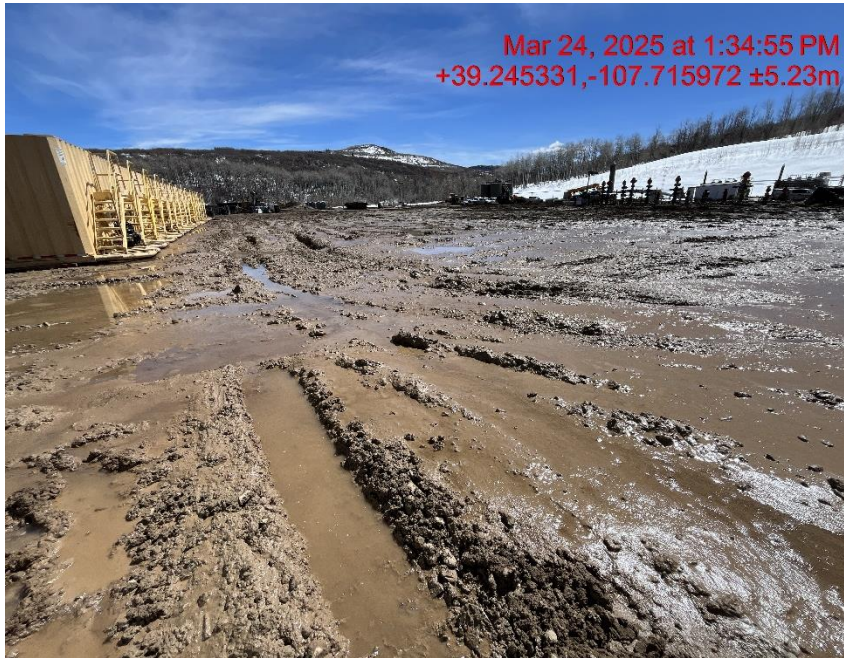
Photo # 6710 Lack of stabilization/compaction on location/insufficient tracking BMP's
