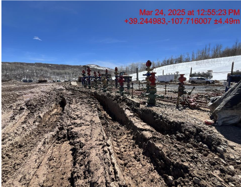
Photo # 6688 Lack of stabilization/compaction on location/insufficient tracking BMP's
