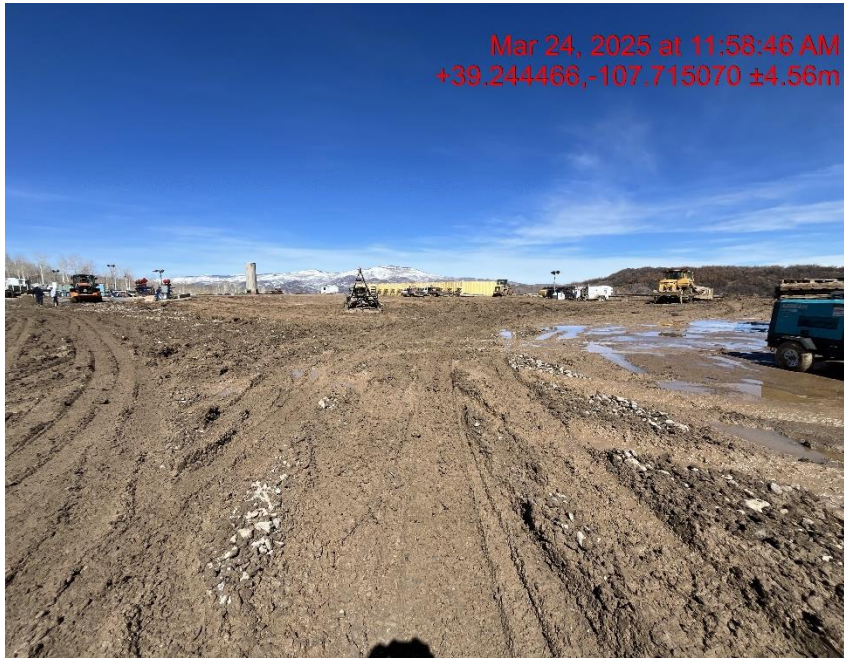
Photo # 6683 Lack of stabilization/compaction on location/insufficient tracking BMP's
