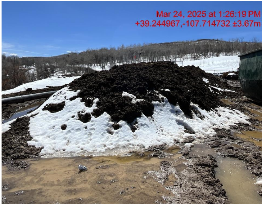
Photo # 6699 Stockpiled soils on location with no BMP's
